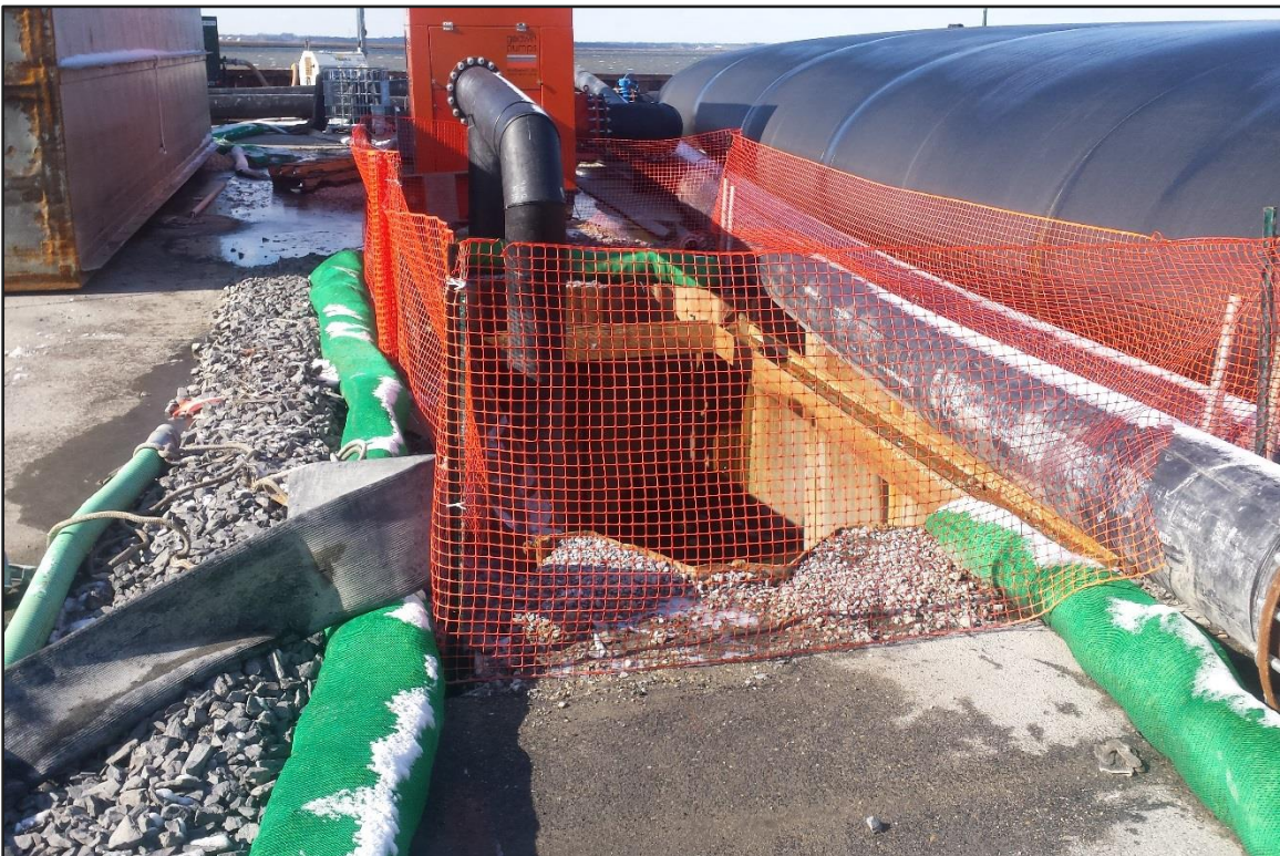
Photograph 8: De-watering Area – Sump pump on standby (Looking west)
