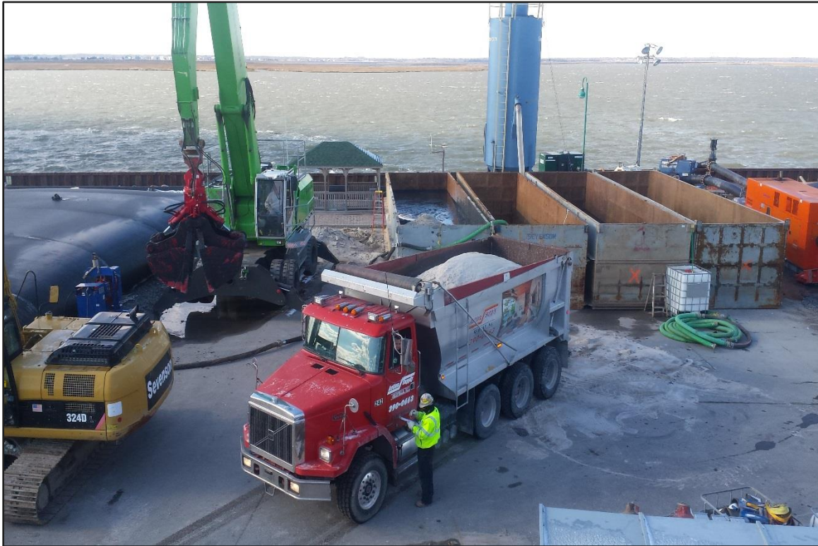
Photograph 9: De-watering Area – Truck delivering sand for blending operations. (Looking west)
