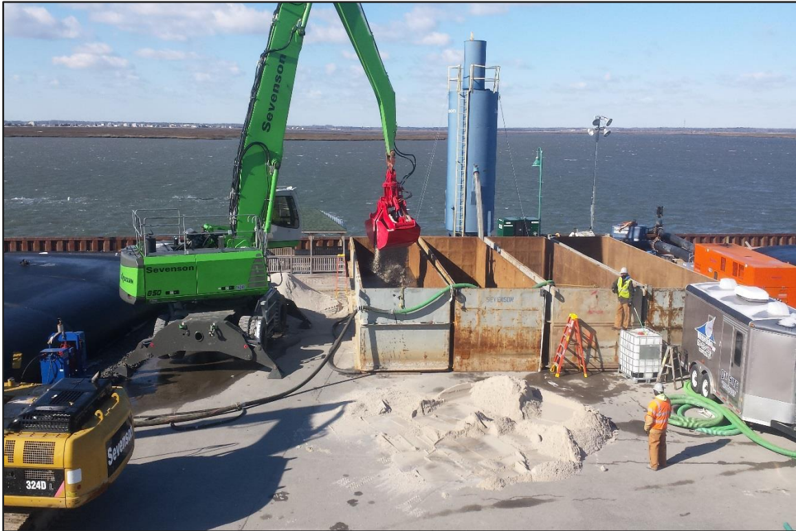
Photograph 5: De-watering Area – Blending sand with dredge material. (Looking west)
