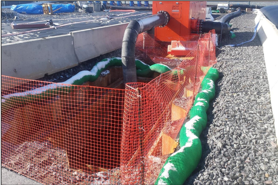
Photograph 11: De-watering Area – Sump pump on standby. (Looking southwest)
