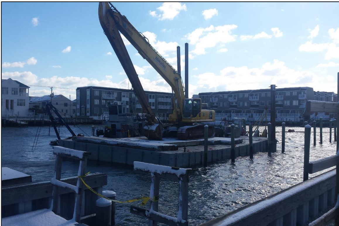
Photograph 6: North Basin – Hydraulic and mechanical dredges on standby. (Looking southeast)
