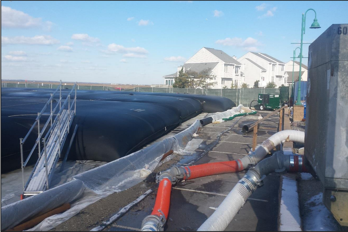
Photograph 7: De-watering Area – Geobags. (Looking northwest)
