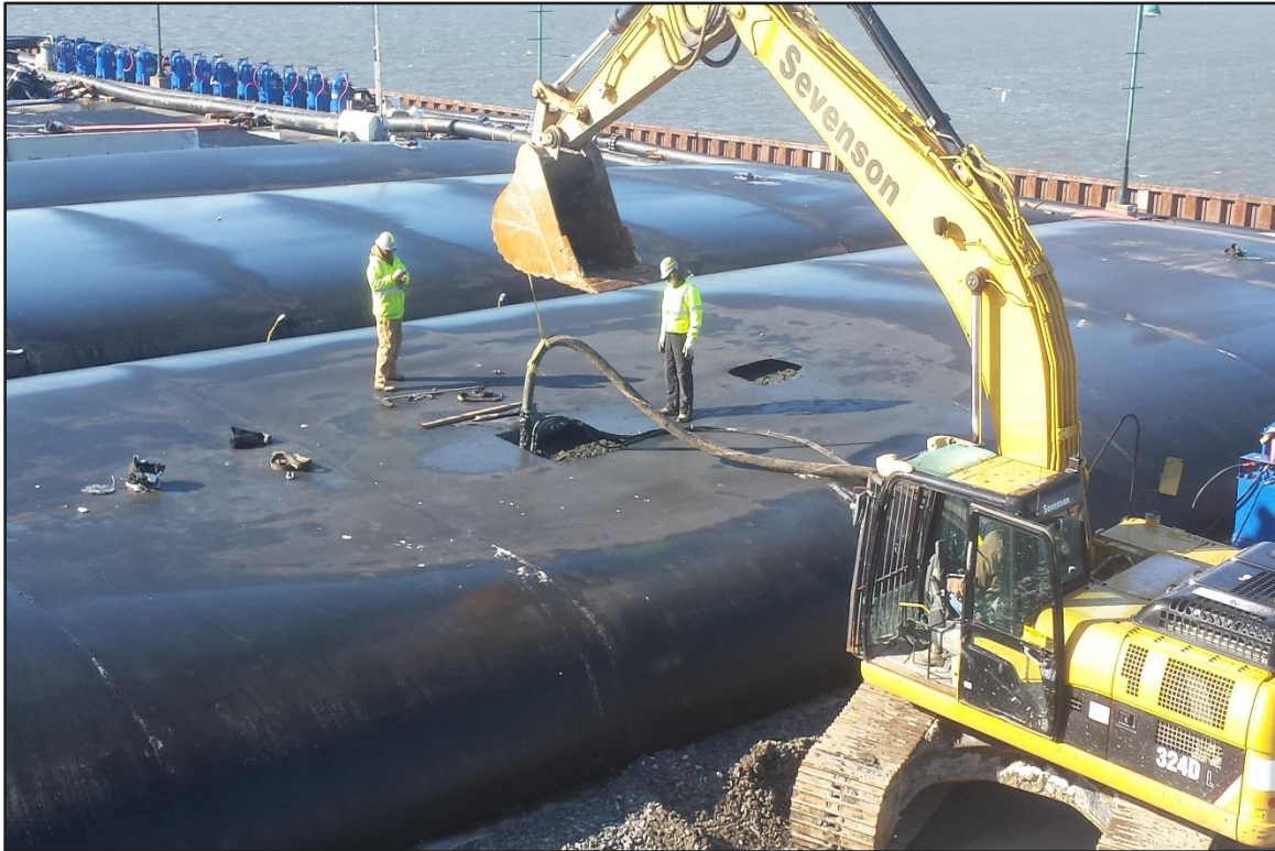
Photograph 3: De-watering Area – Pumping operations after approx. 1 hr. (Looking southwest)
