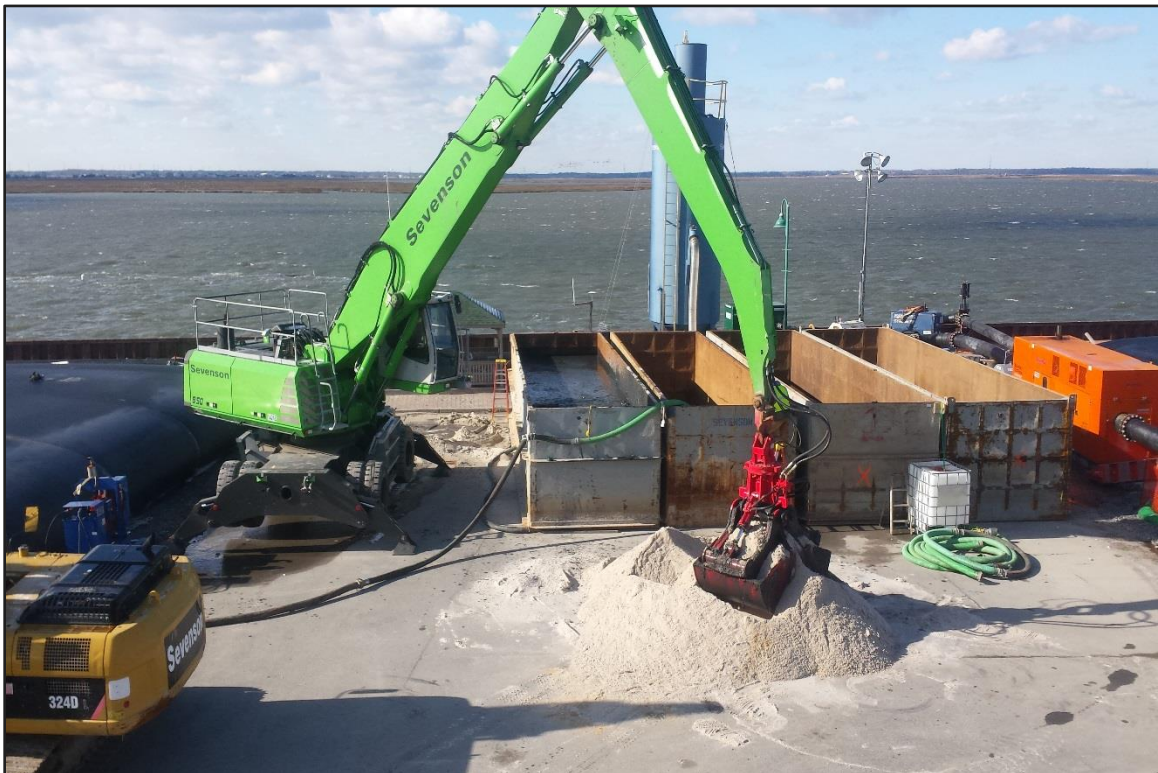
Photograph 14: De-watering Area – Sand blending operations. (Looking west)
