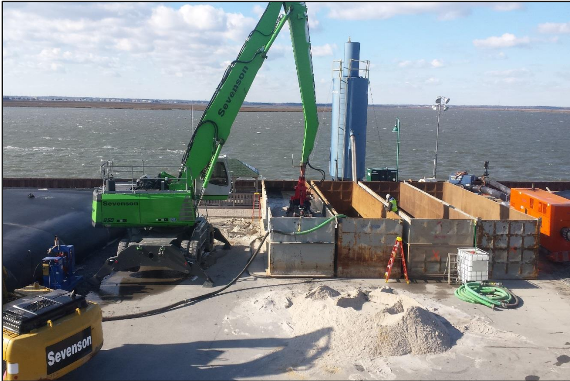
Photograph 15: De-watering Area – Sand blending operations. (Looking west)
