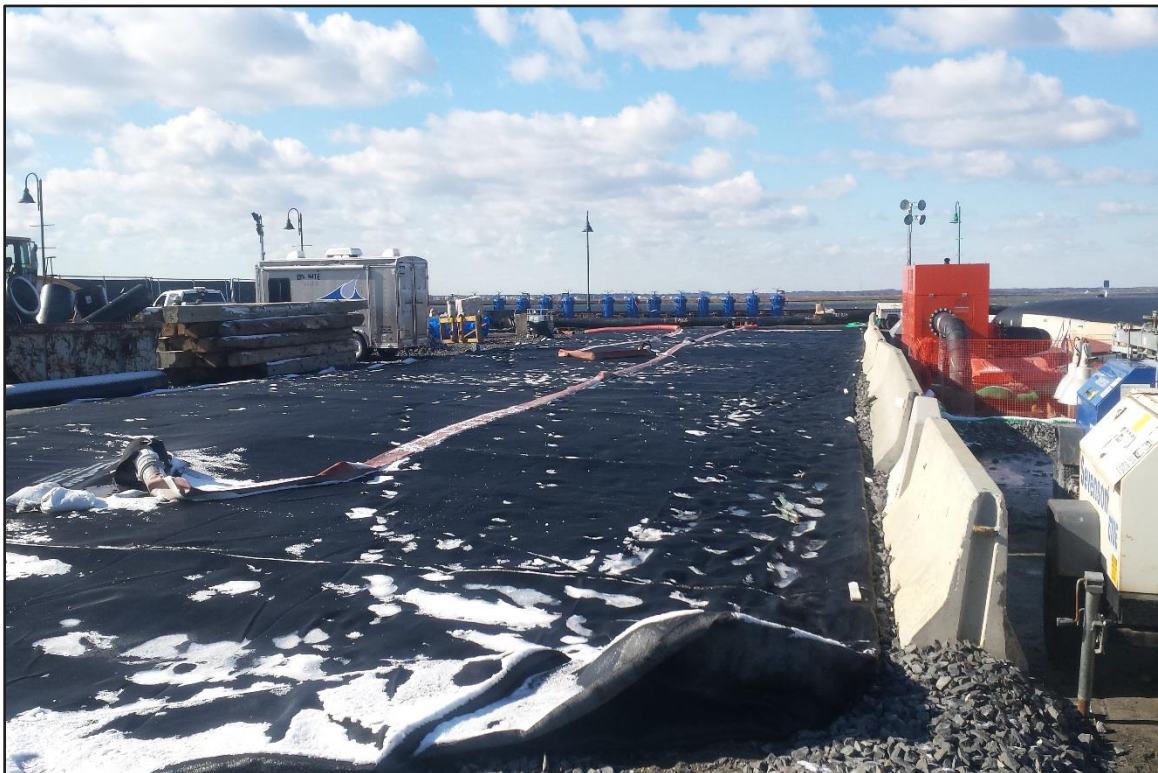
Photograph 12: De-watering Area – Geotube. (Looking west)
