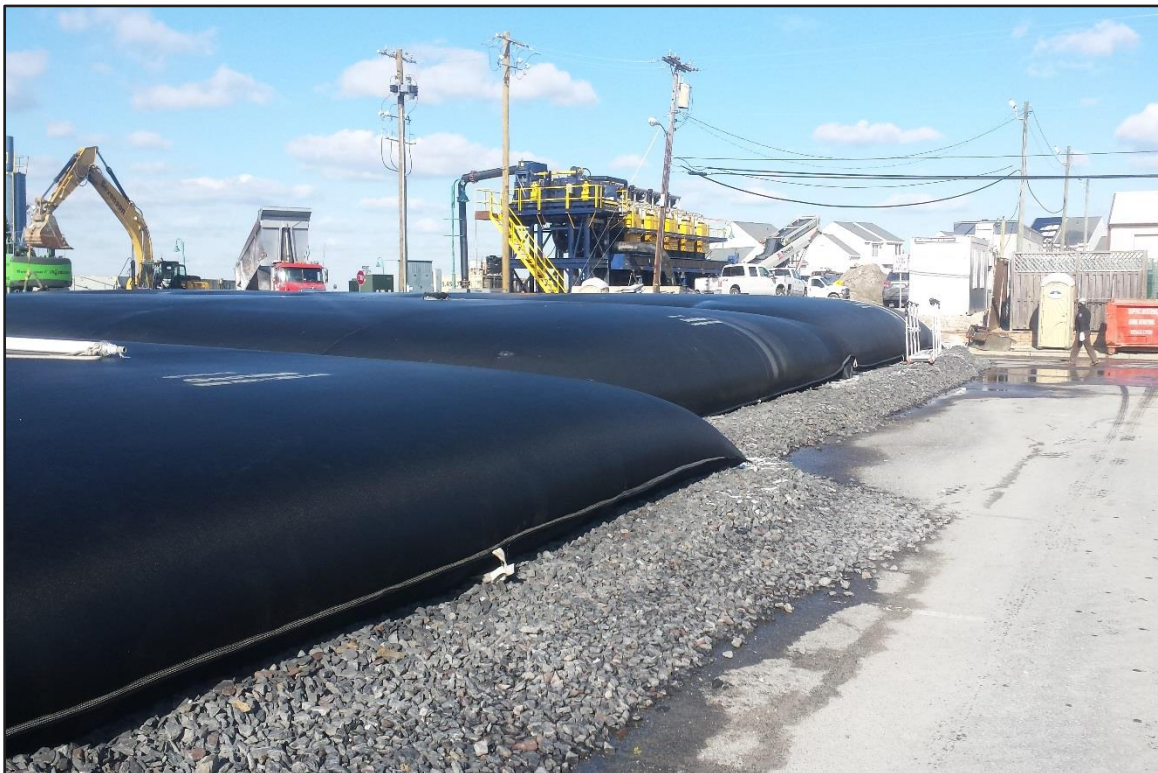
Photograph 10: Geobags. (Looking northwest)
