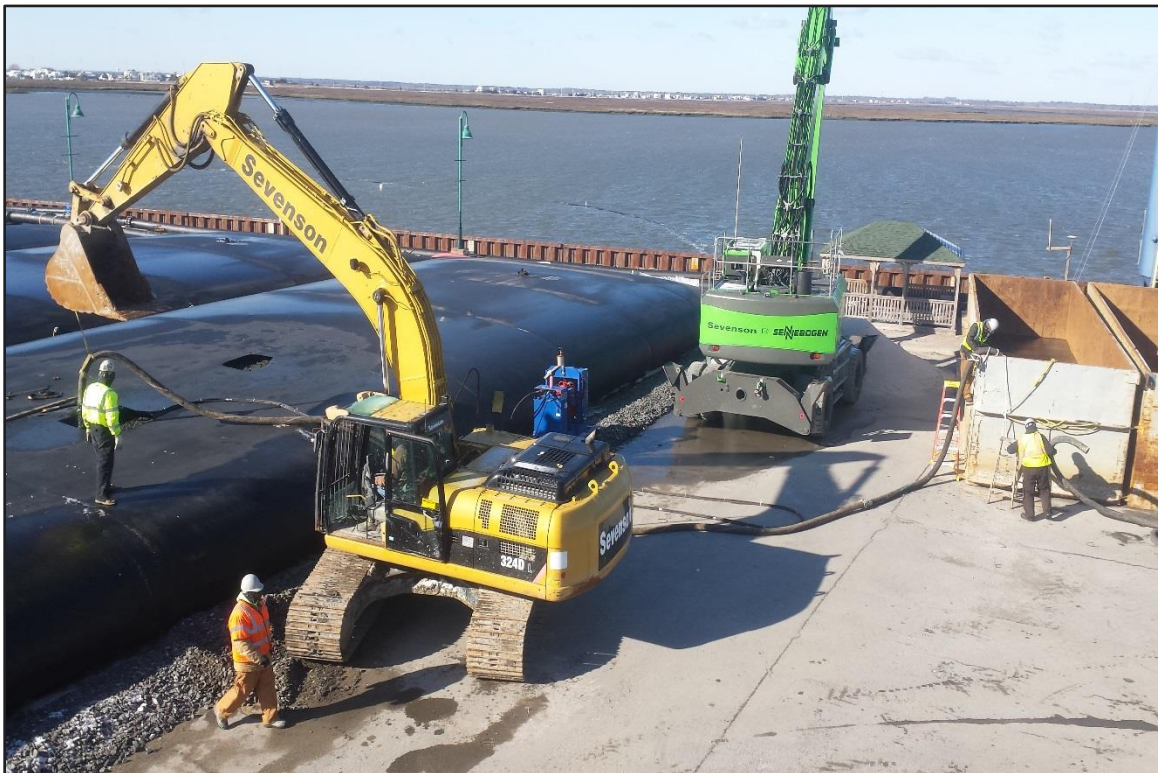
Photograph 2: De-watering Area – Pumping operations after approx. 1 hr. (Looking west)
