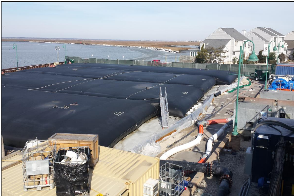
Photograph 14: De-watering area – Geobags on standby. (Looking northwest)
