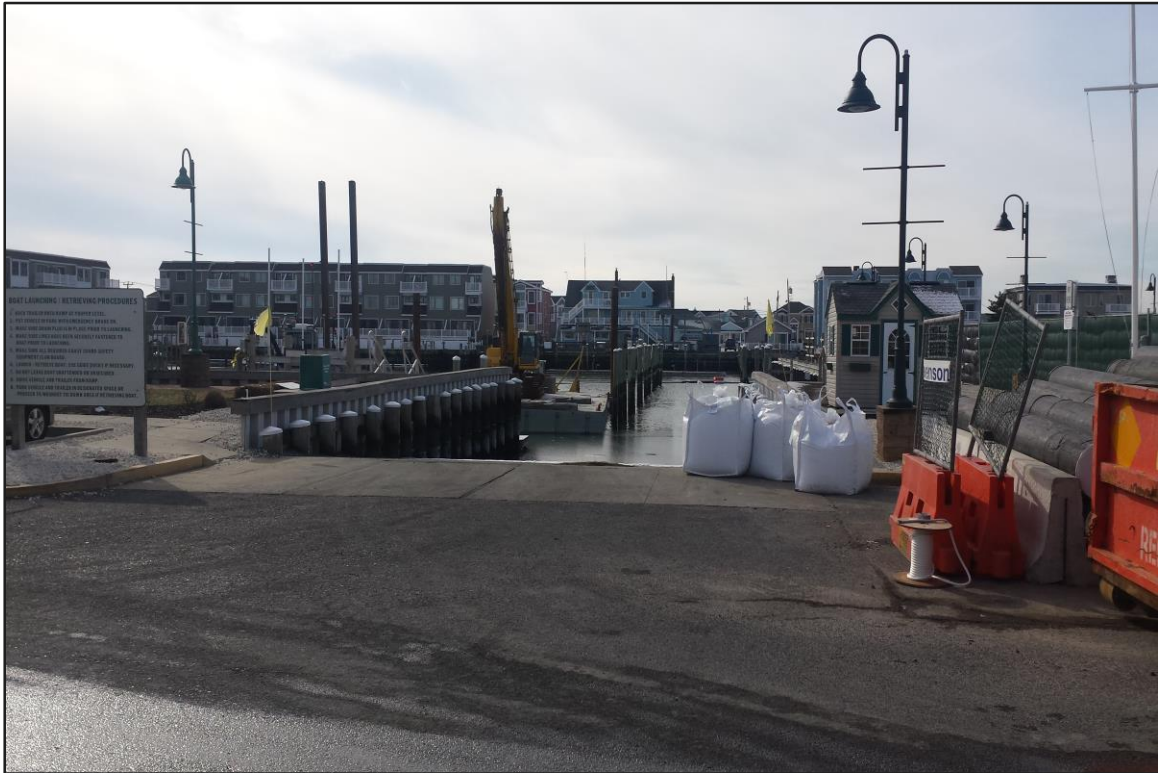
Photograph 3: De-watering area – Sand bags to block storm surge. (Looking south)
