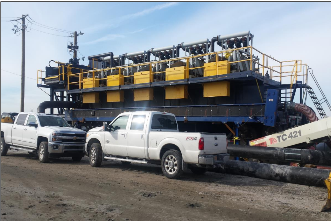
Photograph 2: De-watering area – De-sanding plant on standby. (Looking west)
