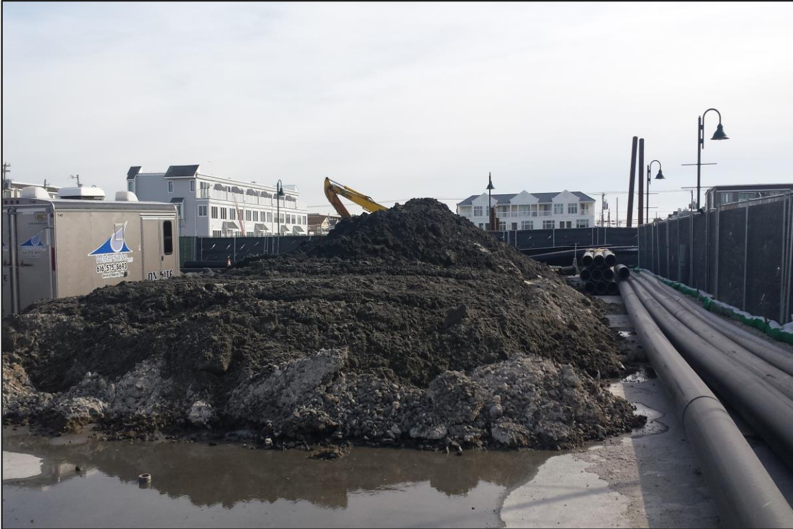
Photograph 9: De-watering area – Blended material staged for removal. (Looking east)
