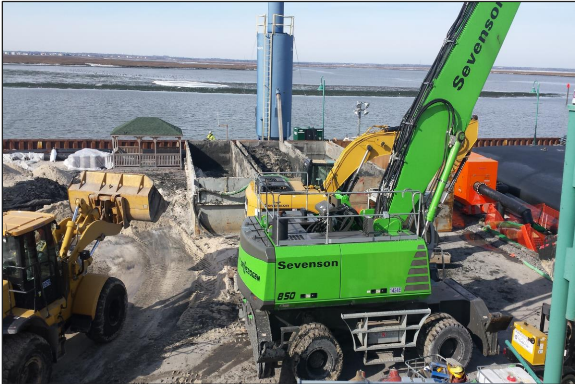
Photograph 13: De-watering area – Sand-blending operations in progress. (Looking west)
