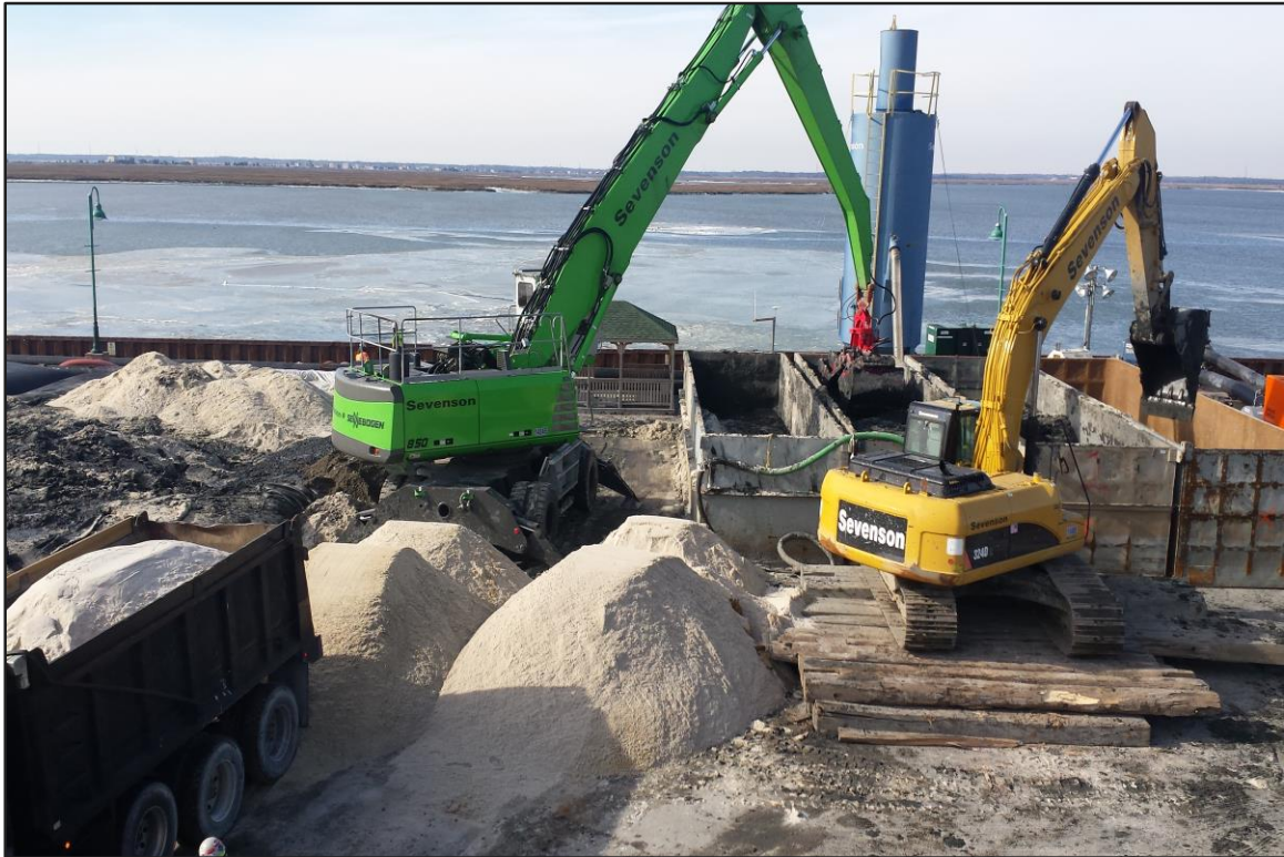
Photograph 17: De-watering area – Sand-blending operations in progress. (Looking west)
