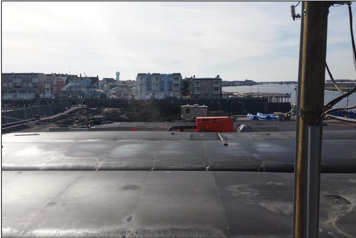
Photograph 15: De-watering area – Blended material staged for removal. (Background, Looking south)
