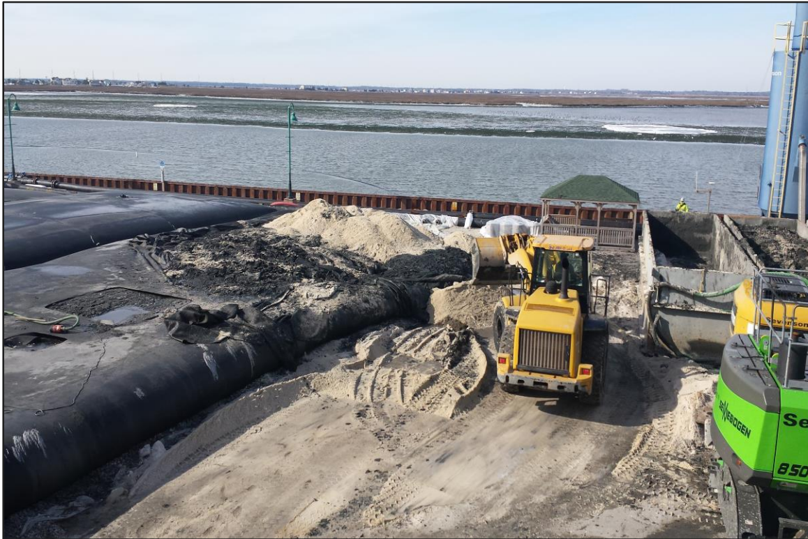
Photograph 11: De-watering area – Sand-blending operations in progress. (Looking west)
