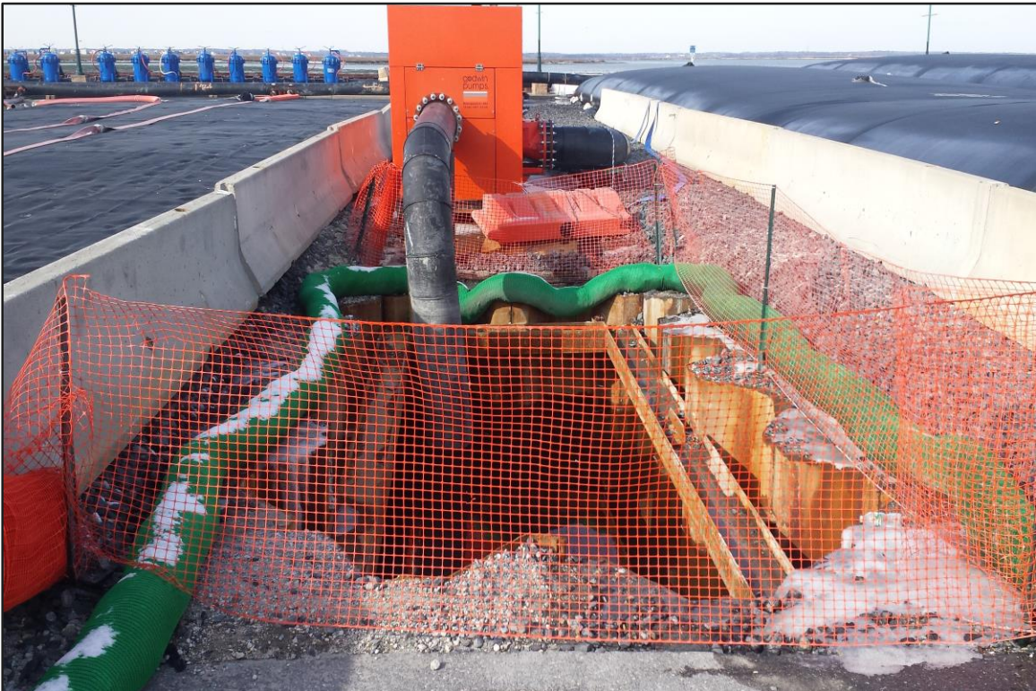
Photograph 10: De-watering area – Sump pump on standby. (Looking west)
