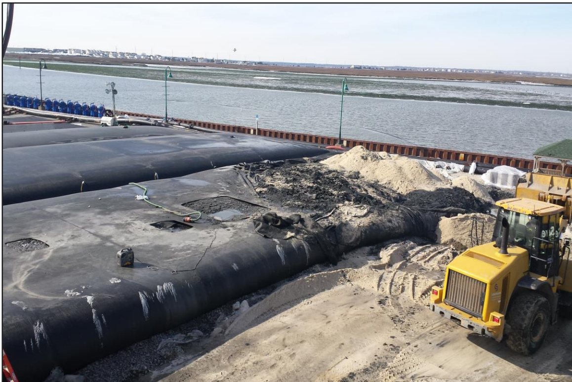
Photograph 12: De-watering area – Sand-blending operations in progress. (Looking southwest)
