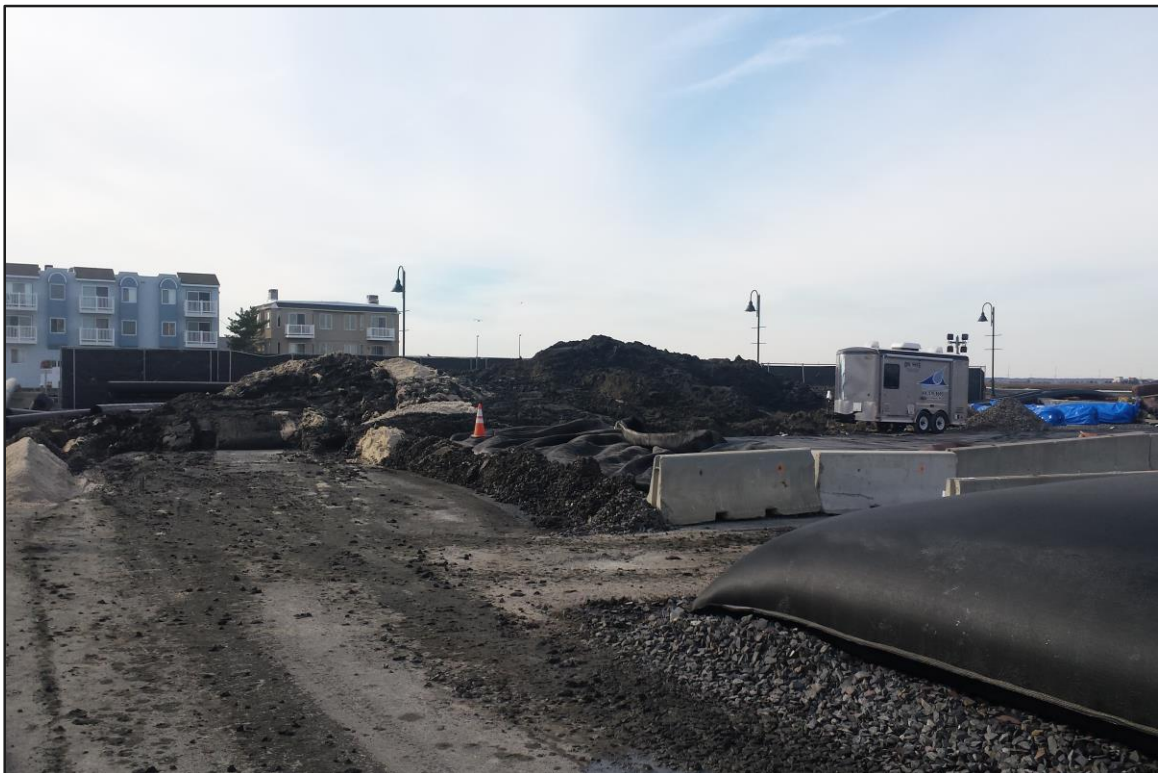
Photograph 4: De-watering area – Blended material staged for removal. (Looking southwest)
