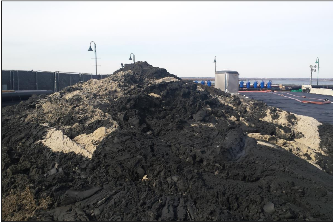
Photograph 5: De-watering area – Blended material staged for removal. (Looking west)
