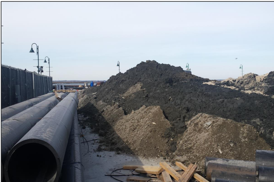
Photograph 6: De-watering area – Blended material staged for removal. (Looking west)
