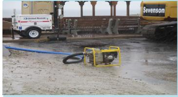
Pumping water from a low elevation on the process pad to Great Channel.
