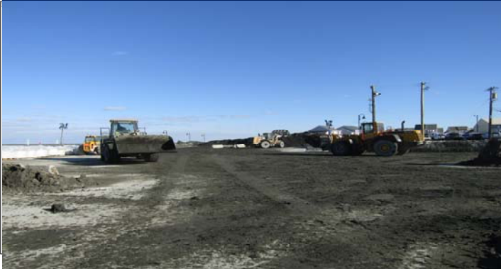
1 Loaders working on the pad moving material
