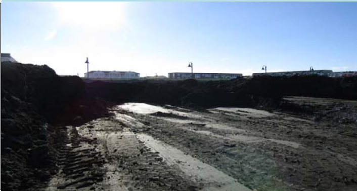
3 Dredge material in staging cell on South pad
