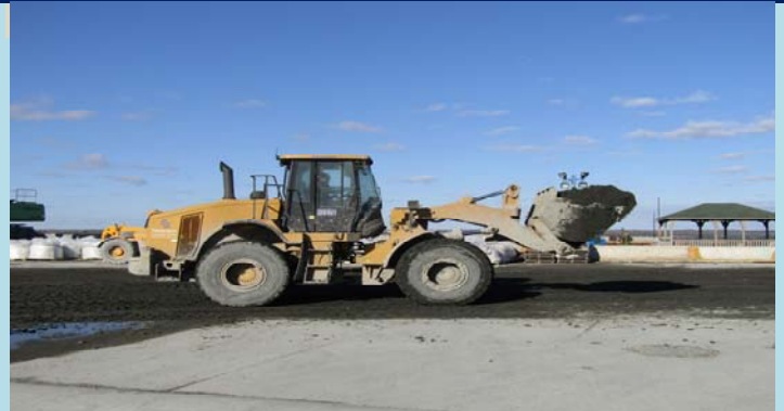
2 Moving ammended dredge material to North pad
