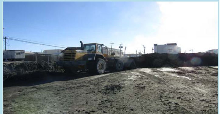
4 Loader clearing material from South pad staging cell
