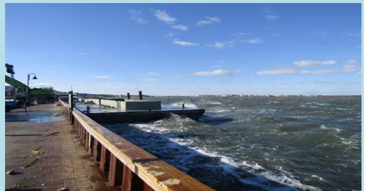
6 Scows secured at the wall for high winds
