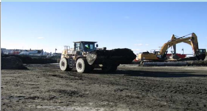
5 Loader moving ammended dredge material for further drying
