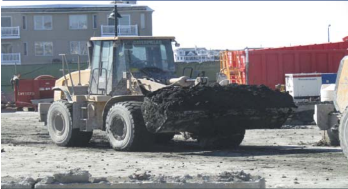
1 Transporting ammended dredge material during load out activities
