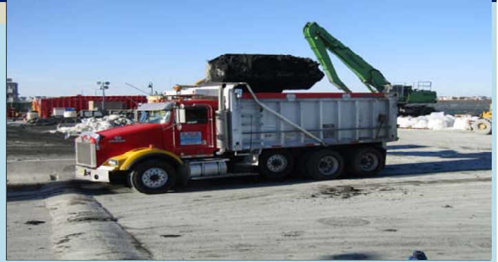
2 Loading material for off-site disposal
