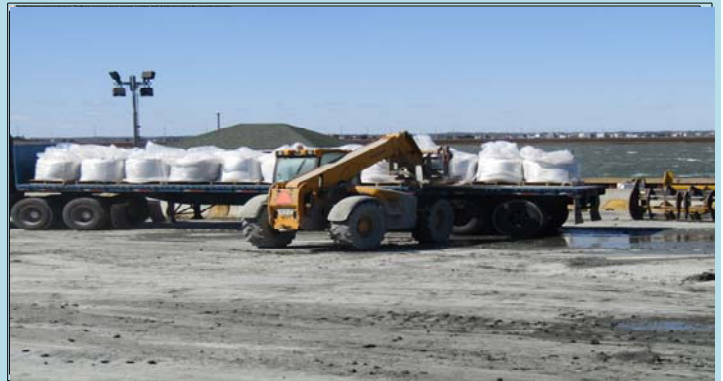
4 Offloading portland cement at the mixing area on the pad
