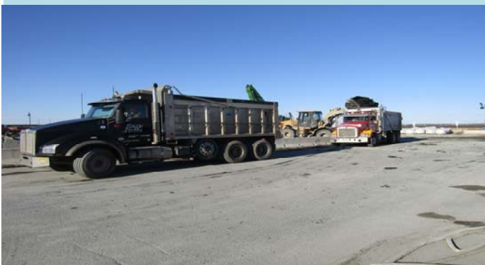
5 Tri-axle dump trucks leaving the jobsite
