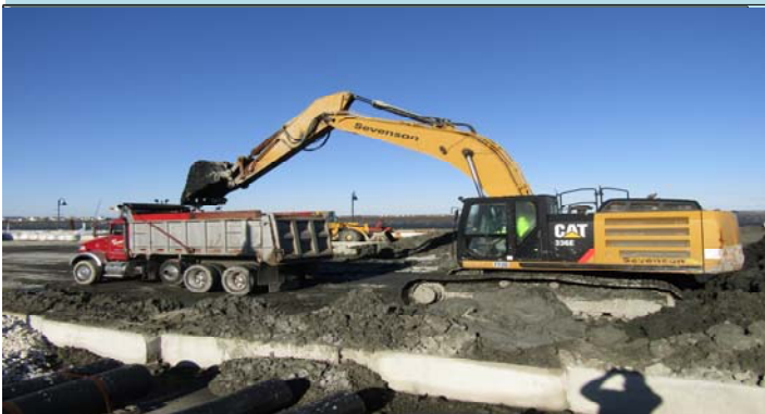
3 Using an excavator to load out dredge material
