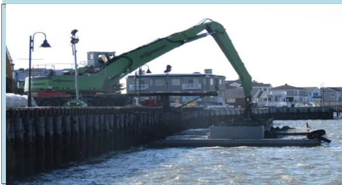
5 Sennebogen unloading a scow at the bulkhead
