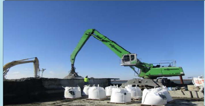
4 Mixing dredged material with Portland cement
