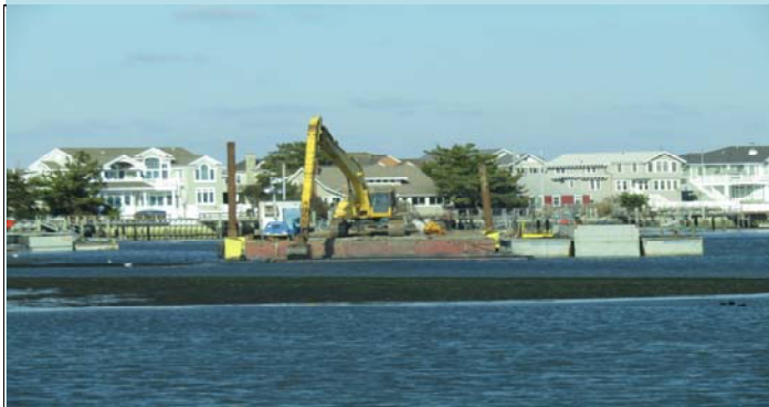
3 PC-400 longfront dredging in the Access Channel at low tide
