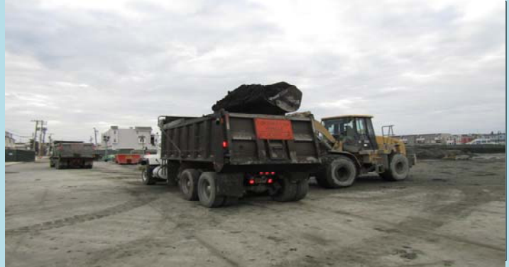
4 Loading a truck with ammended dredge material
