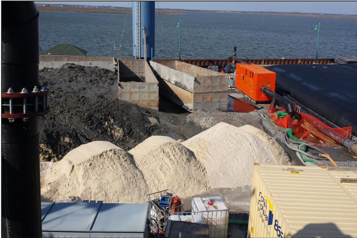
Photograph 3: De-watering Area – Sand for blending, mixing boxes, sump pump on standby. (Looking west)
