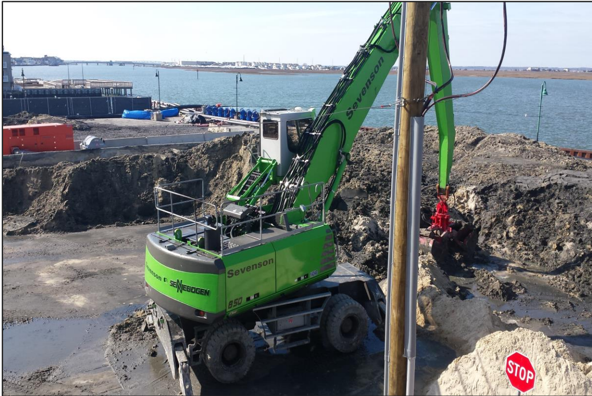
Photograph 5: De-watering Area – Sand blending and removal operations. (Looking southwest)
