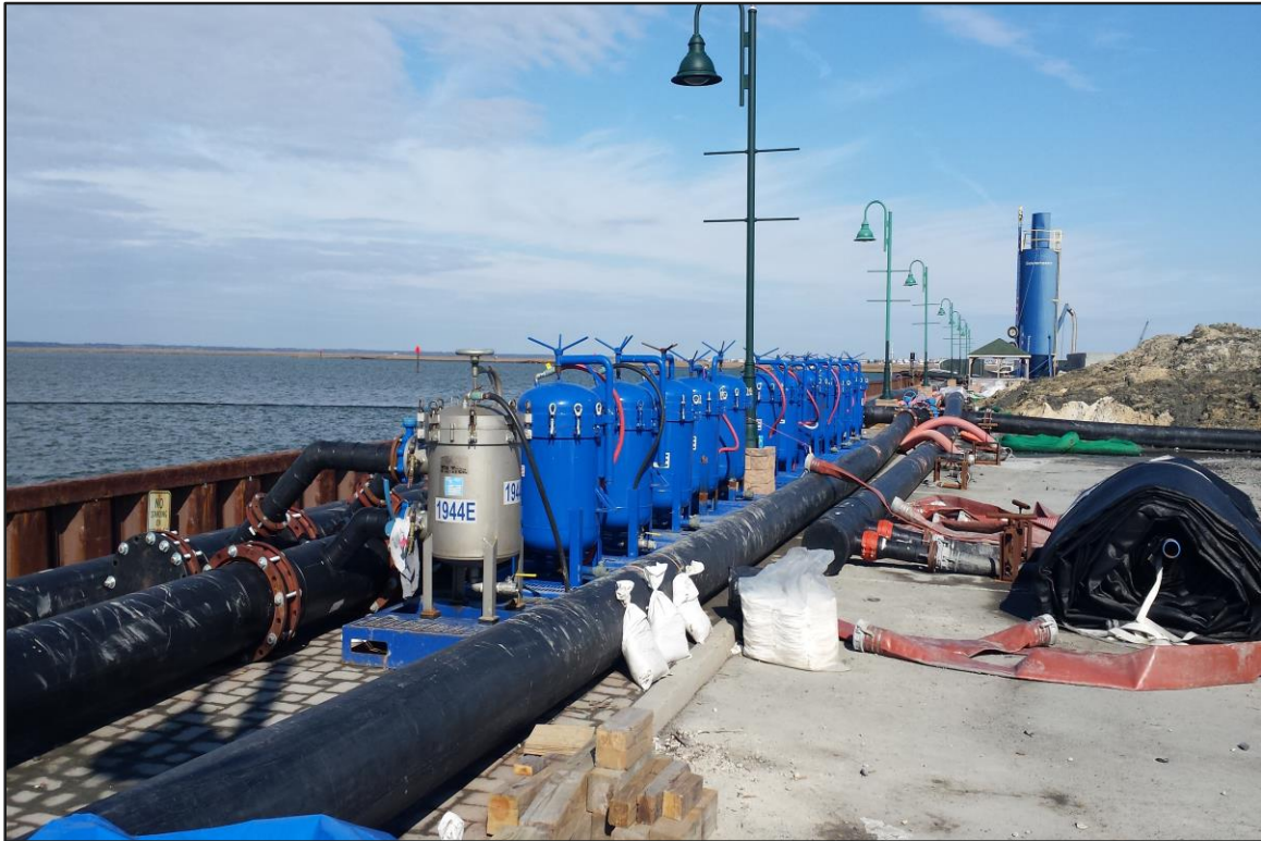
Photograph 13: De-watering Area – Filtration system on standby. (Looking north)
