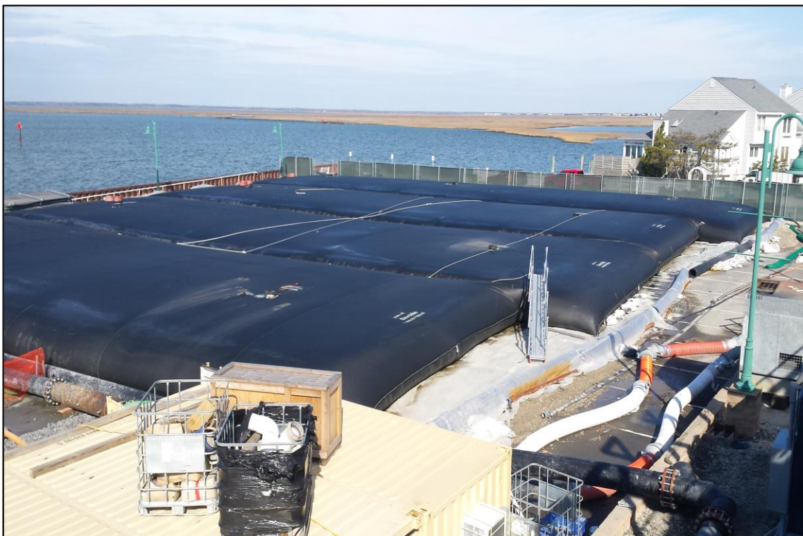
Photograph 2: De-watering Area – Geobags #6-9 on standby. (Looking northwest)
