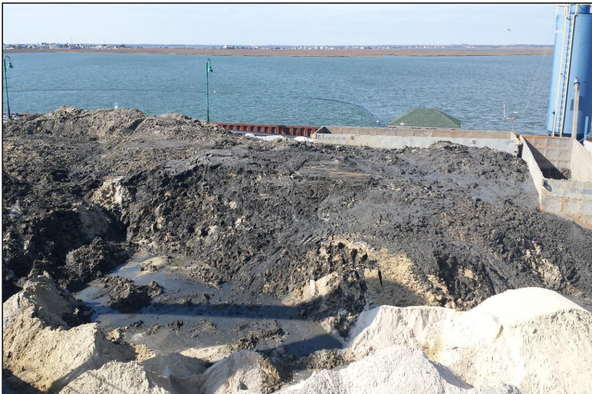
Photograph 4: De-watering Area – Blended material ready for removal. (Looking west)
