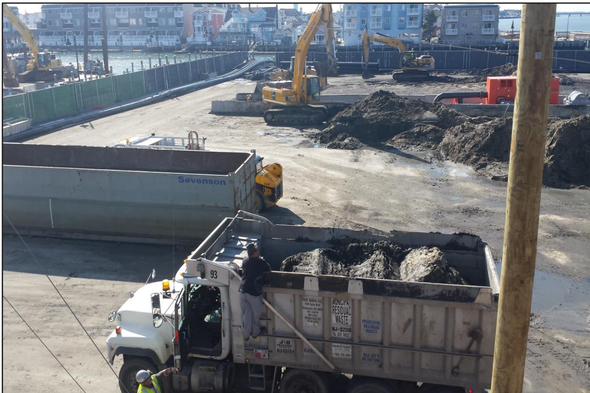
Photograph 6: De-watering Area – Sand blending and removal operations. (Looking south)
