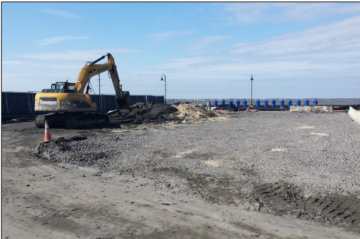
Photograph 10: De-watering Area – Sand blending operations alongside a prepared de-watering pad. (Looking west)
