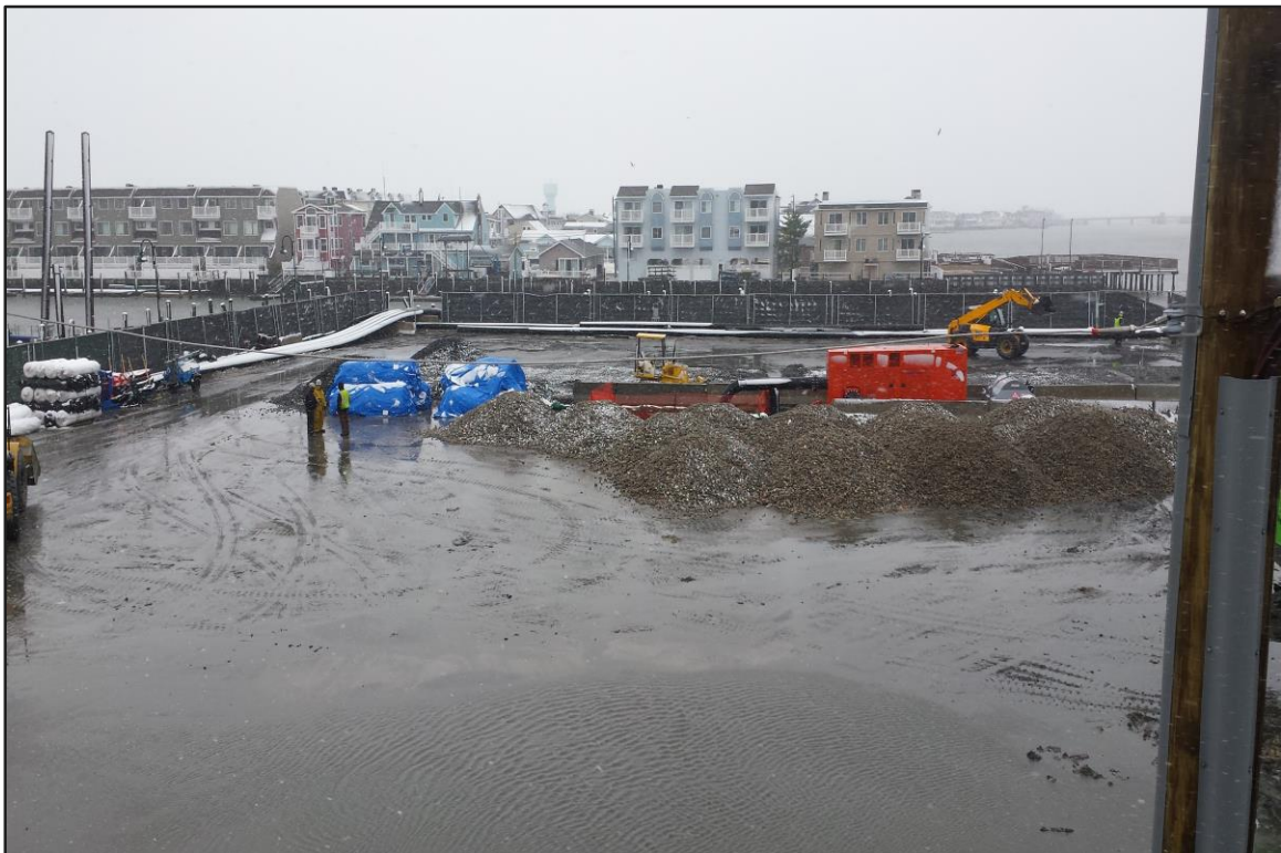
Photograph 6: De-watering Area – Equipment preparing pads for new geobags. (Looking south)
