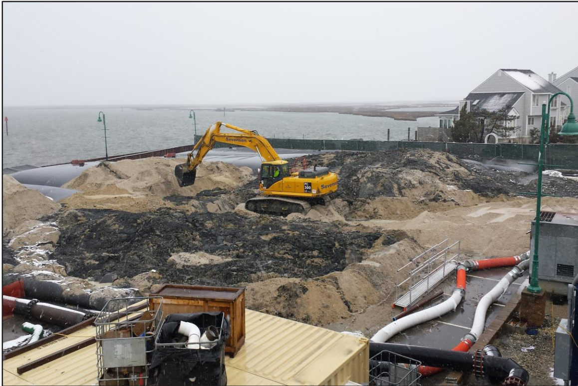
Photograph 3: De-watering Area – Sand blending geobags #6-9. (Looking northwest)
