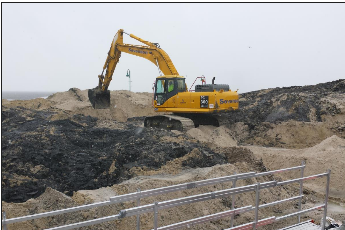
Photograph 10: De-watering Area – Sand blending geobags #6-9. (Looking northwest)
