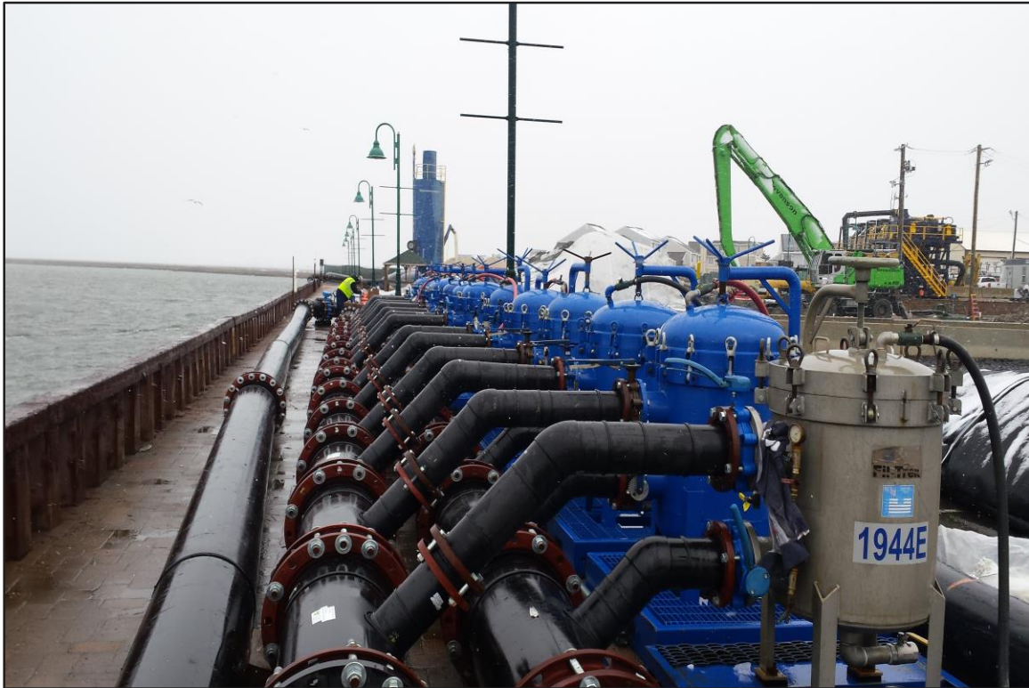
Photograph 9: De-watering Area – Filtration system in operation. (Looking north)
