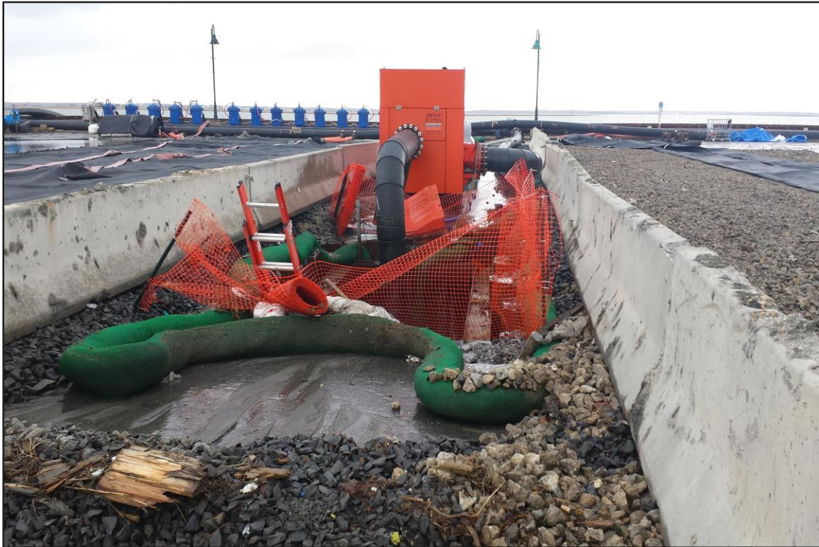
Photograph 9: De-watering Area – Sump pump on standby. (Looking west)
