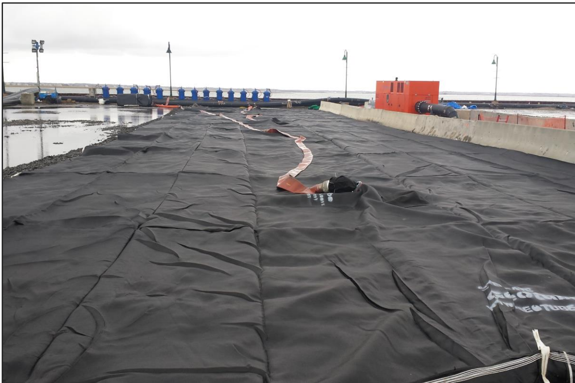
Photograph 10: De-watering Area – New geobag on standby. (Looking west)
