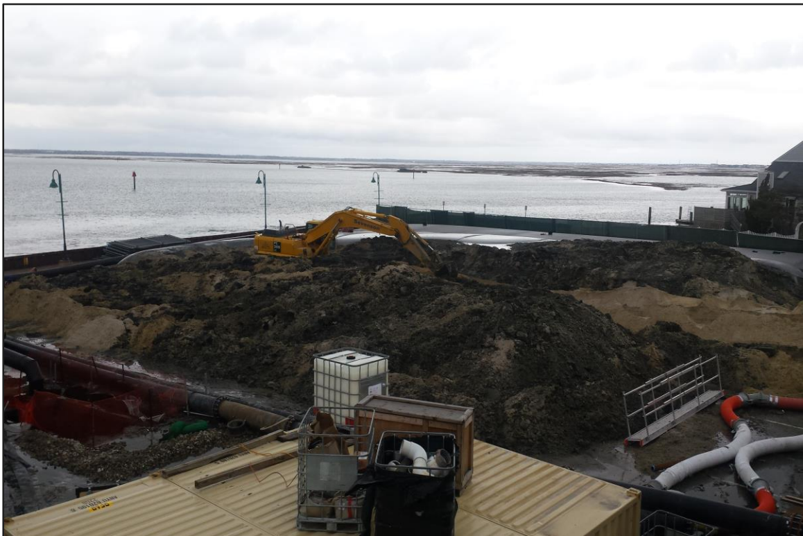
Photograph 6: De-watering Area – Sand blending in progress. (Looking northwest)
