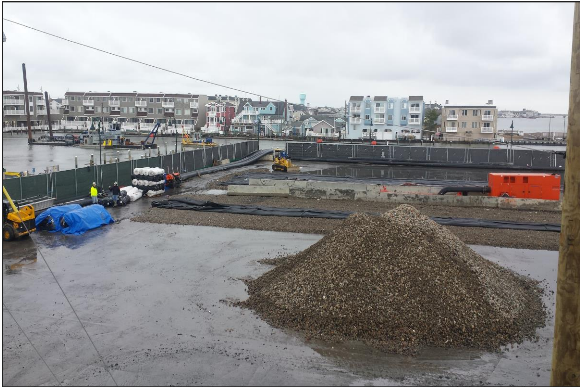
Photograph 3: De-watering Area – Geobag pad preparation in progress. (Looking south)
