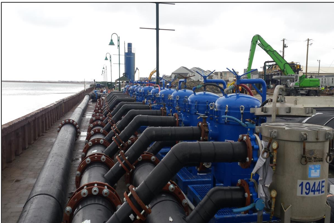
Photograph 12: De-watering Area – Filtration system on standby. (Looking north)
