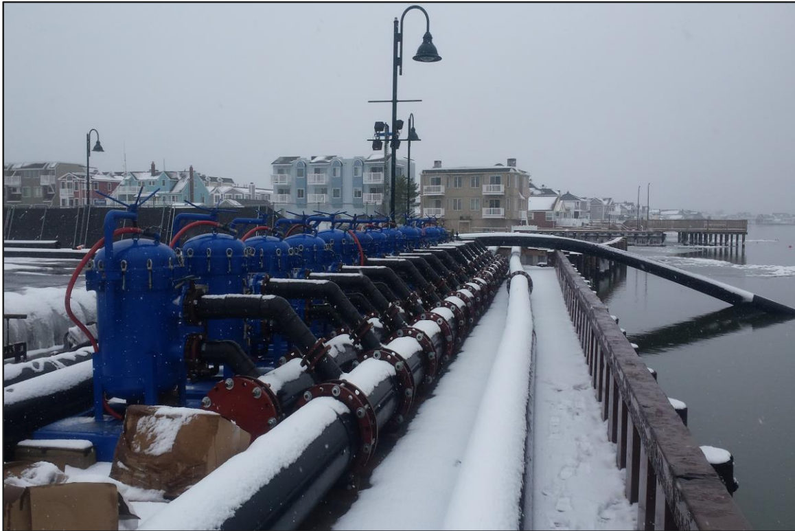
Photograph 7: De-watering area – Filtration system. (Looking south)
