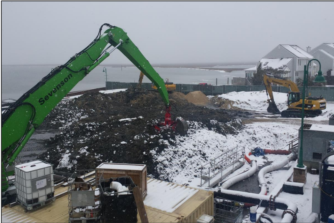
Photograph 5: De-watering Area – Sand blending operations in progress. (Looking northwest)
