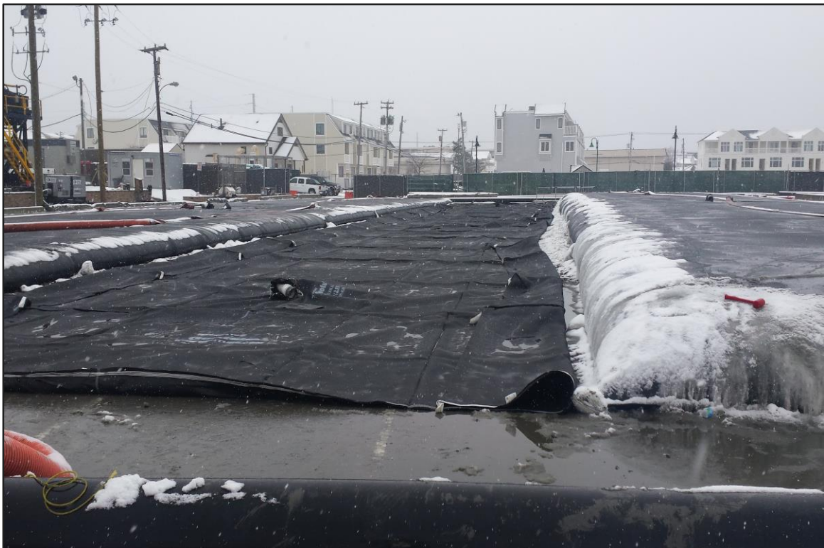
Photograph 6: De-watering Area – Geobag #4. (Looking east)
