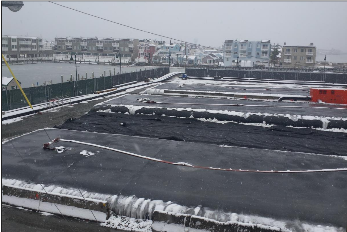
Photograph 3: De-watering Area – Geobags #2-5. (Looking south)
