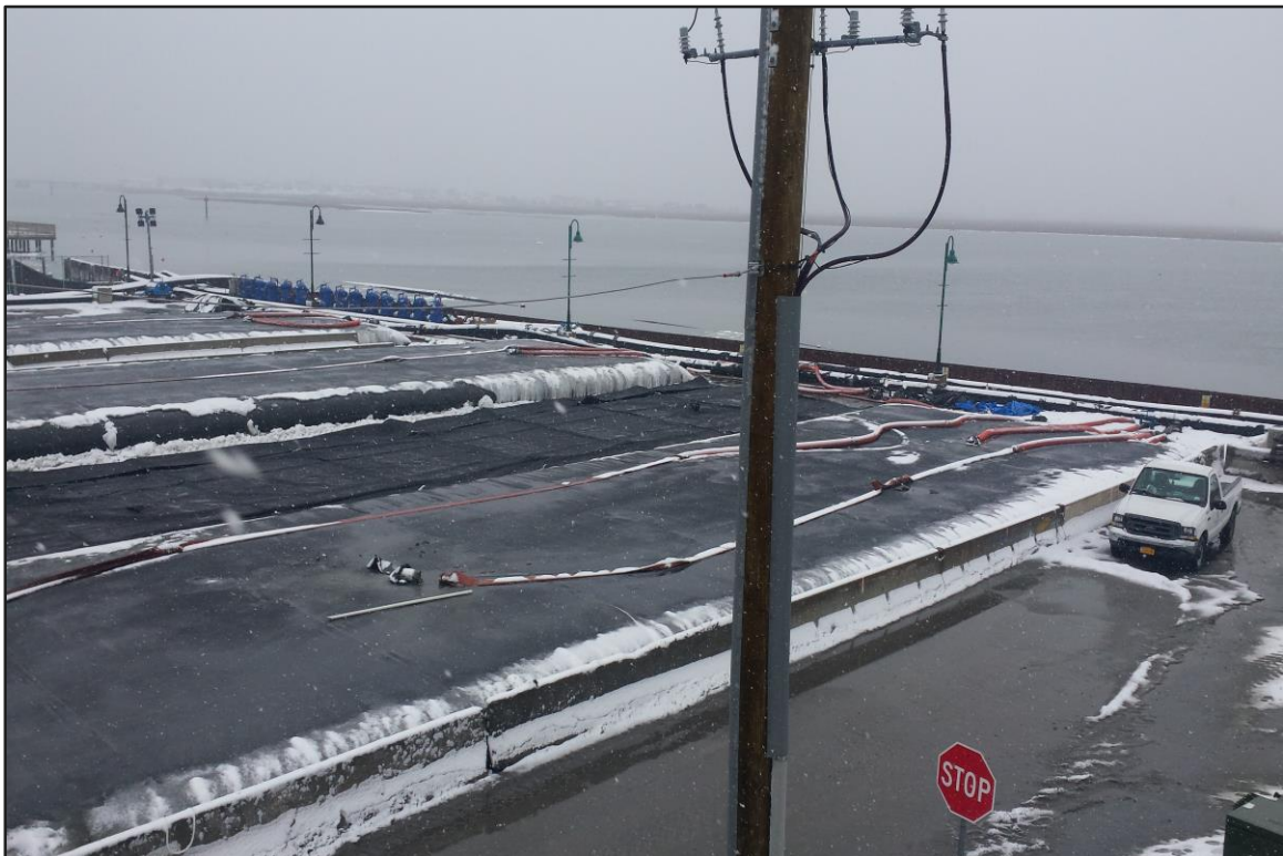
Photograph 4: De-watering Area – Geobags #2-5. (Looking southwest)
