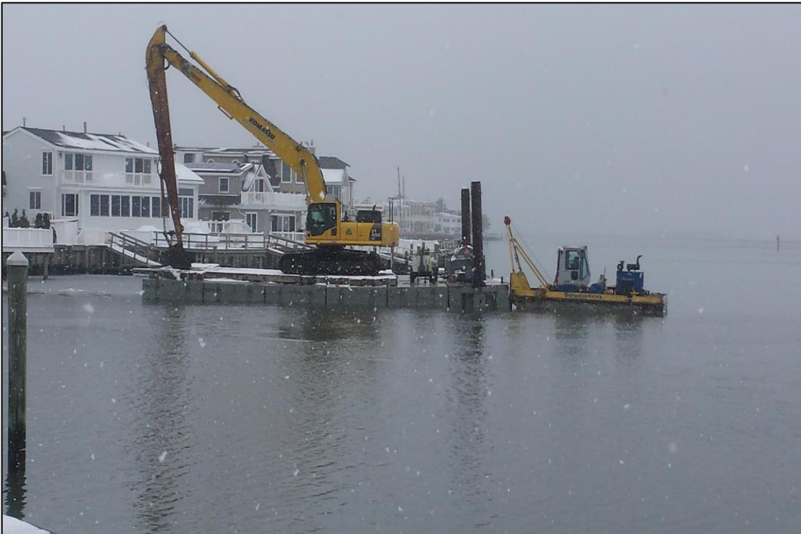
Photograph 10: Shelter Haven – Mechanical dredge. (Looking south)
