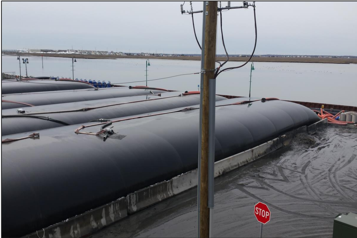
Photograph 7: De-watering Area – Geobags #2-5 in operation. (Looking southwest)
