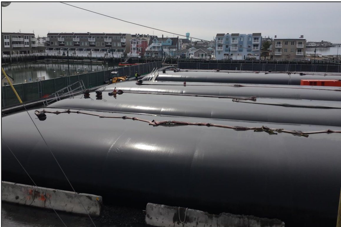
Photograph 6: De-watering Area – Geobags #1-5 in operation. (Looking south)
