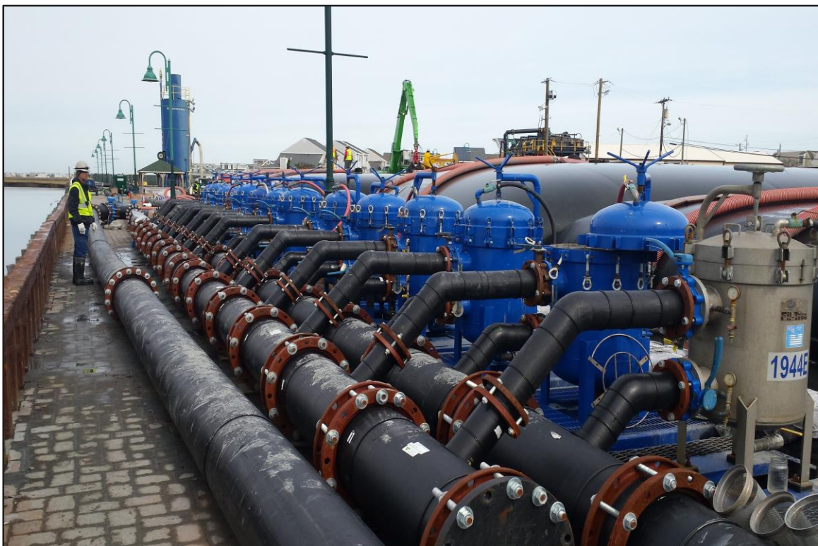
Photograph 12: De-watering Area – Filtration system in operation. (Looking north)
