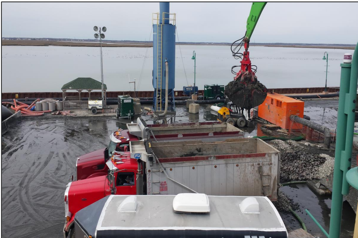
Photograph 8: De-watering Area – Trucks loaded with blended dredge material. (Looking west)
