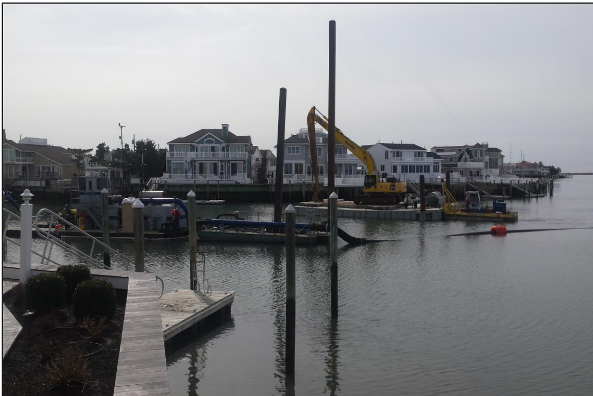
Photograph 2: Shelter Haven – Hydraulic and mechanical dredges. (Looking south)
