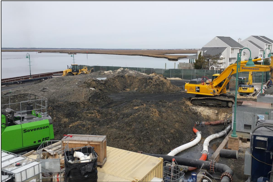
Photograph 9: De-watering Area – Blended dredge material staged for removal. (Looking northwest)
