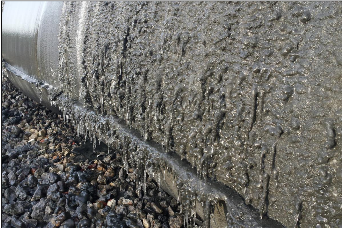
Photograph 1: De-watering Area – Frozen geobag runoff.
