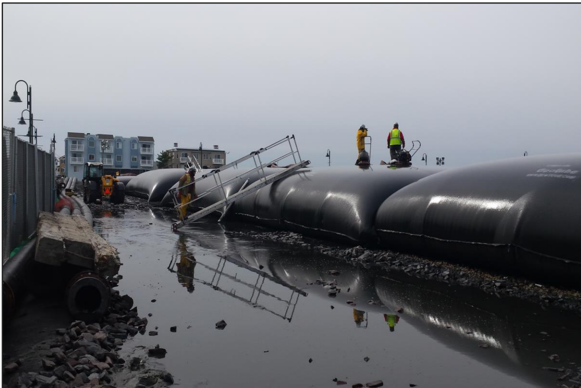
Photograph 10: De-watering Area – Geobags #1-5 in operation. (Looking southwest)
