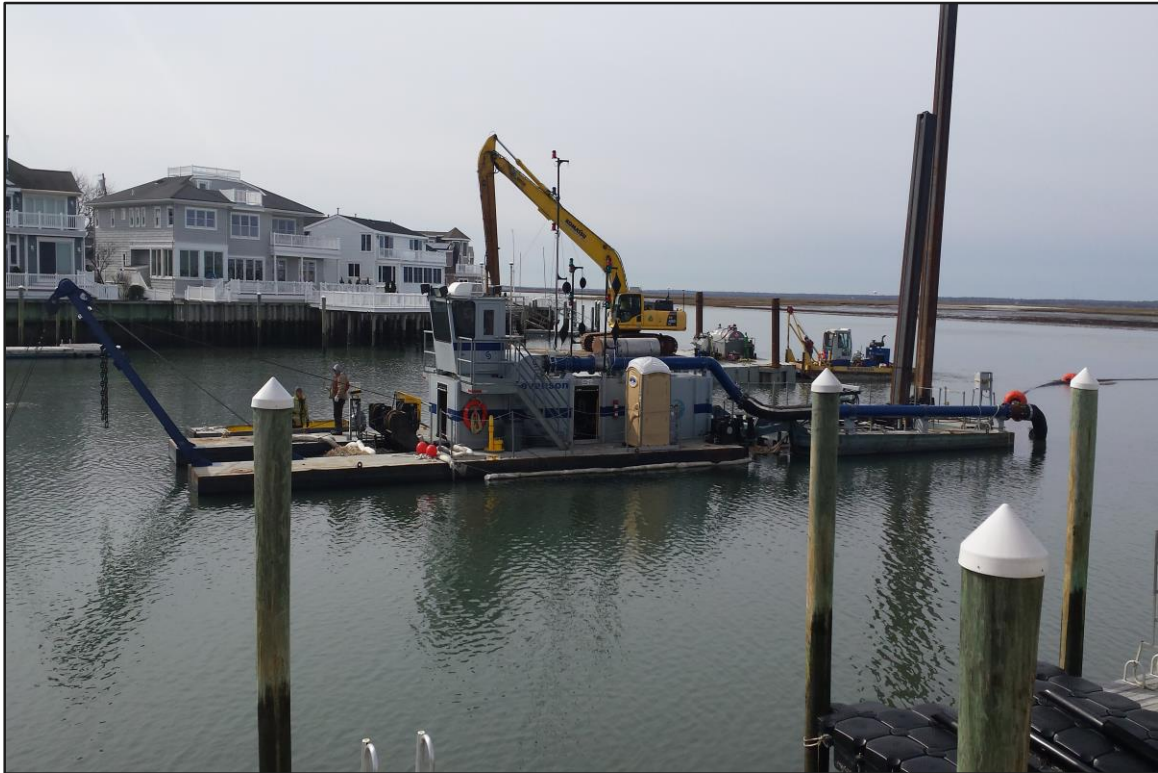
Photograph 3: Shelter Haven – Hydraulic and mechanical dredges. (Looking southwest)
