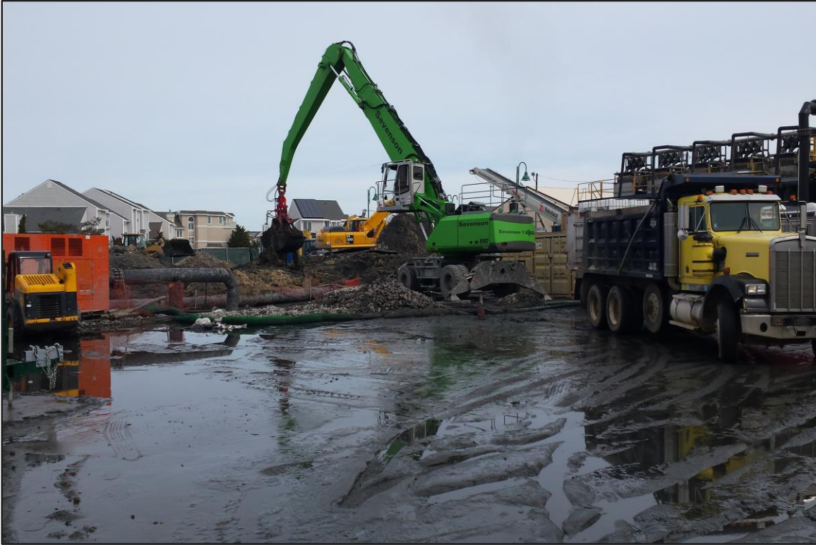
Photograph 13: De-watering Area – Trucks loaded with blended dredge material. (Looking north)
