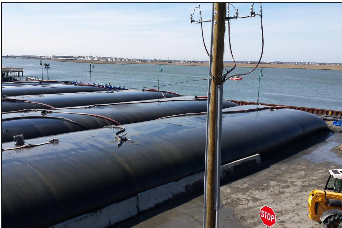
Photograph 6: De-watering Area – Geobags #1-5 in operation. (Looking southwest)
