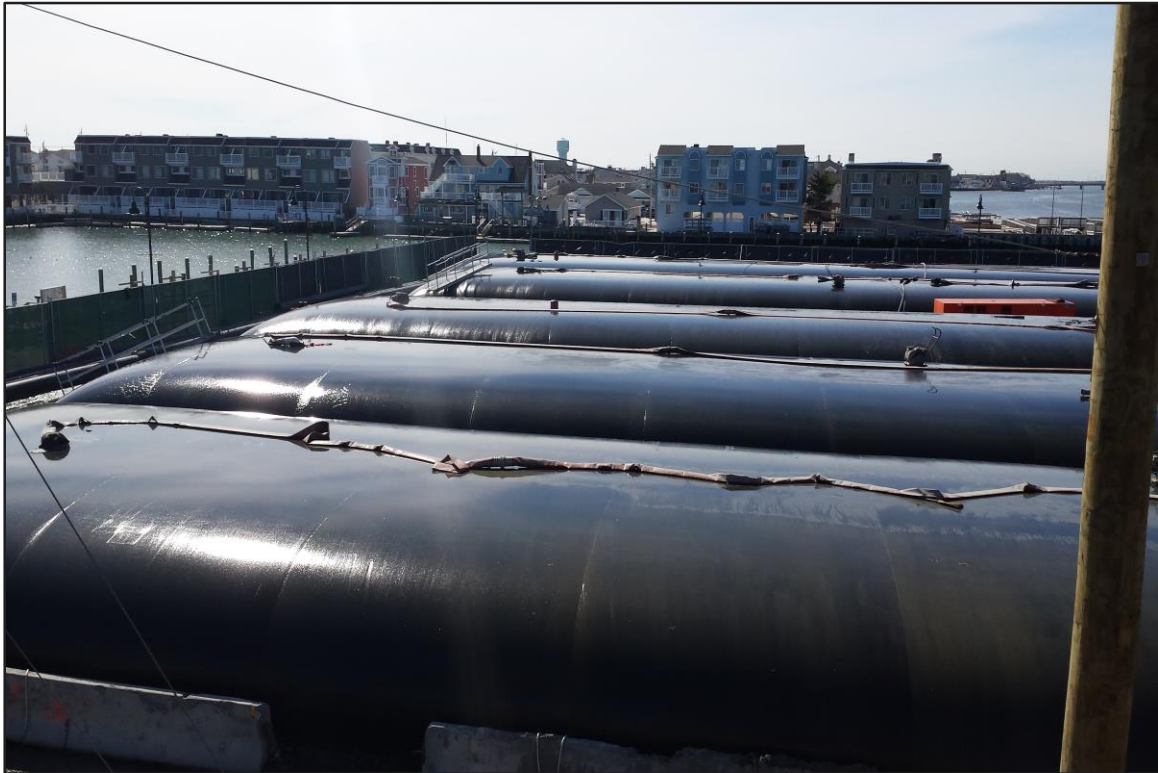
Photograph 5: De-watering Area – Geobags #1-5 in operation. (Looking south)
