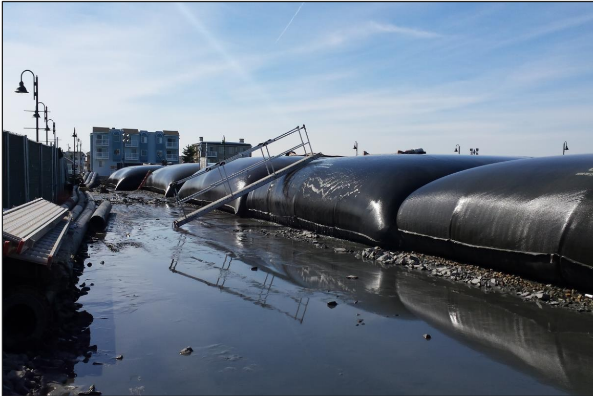
Photograph 9: De-watering Area – Geobags #1-5 in operation. (Looking south)
