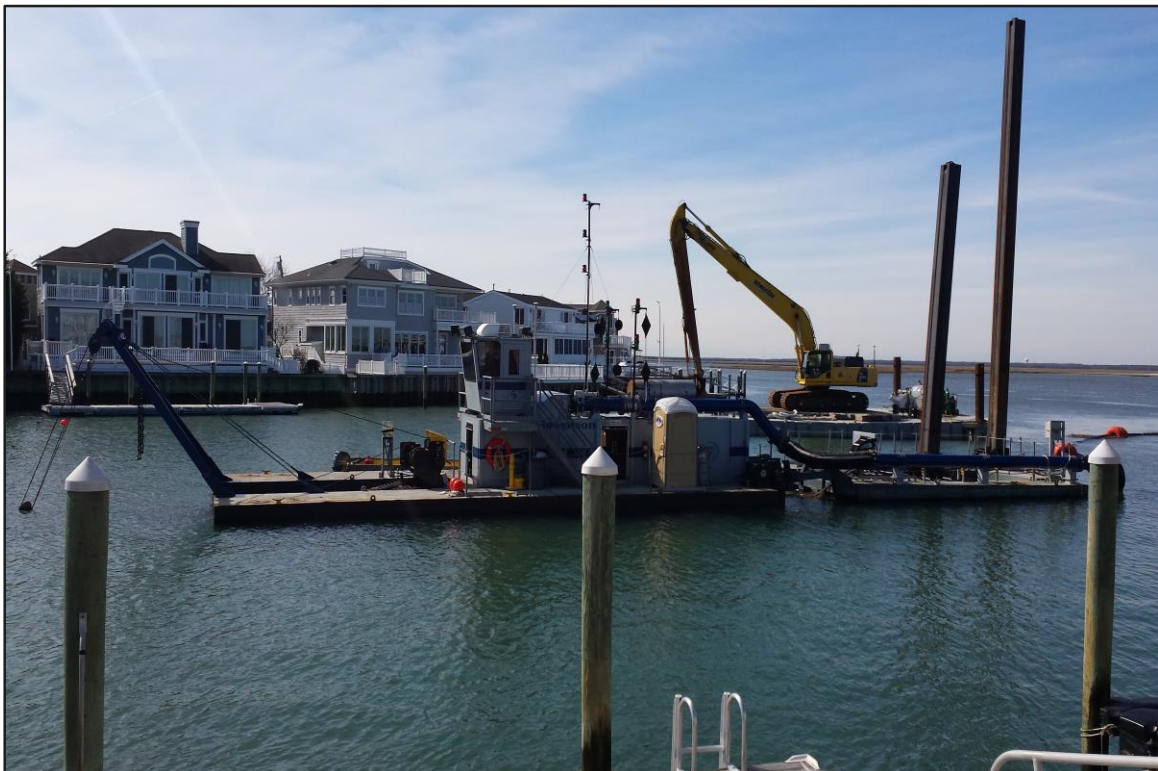
Photograph 2: Shelter Haven - Hydraulic Dredge in operation. (Looking south)
