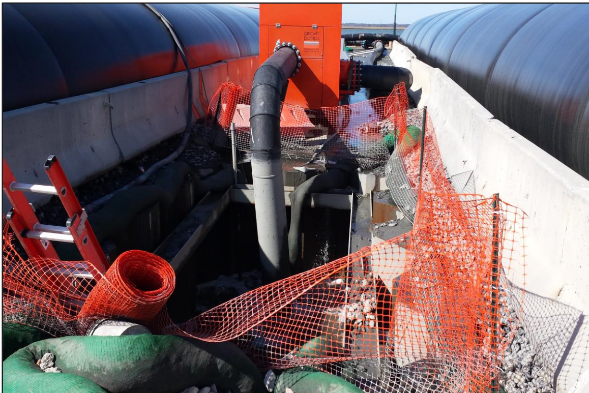
Photograph 10: De-watering Area – Sump pump in operation. (Looking west)
