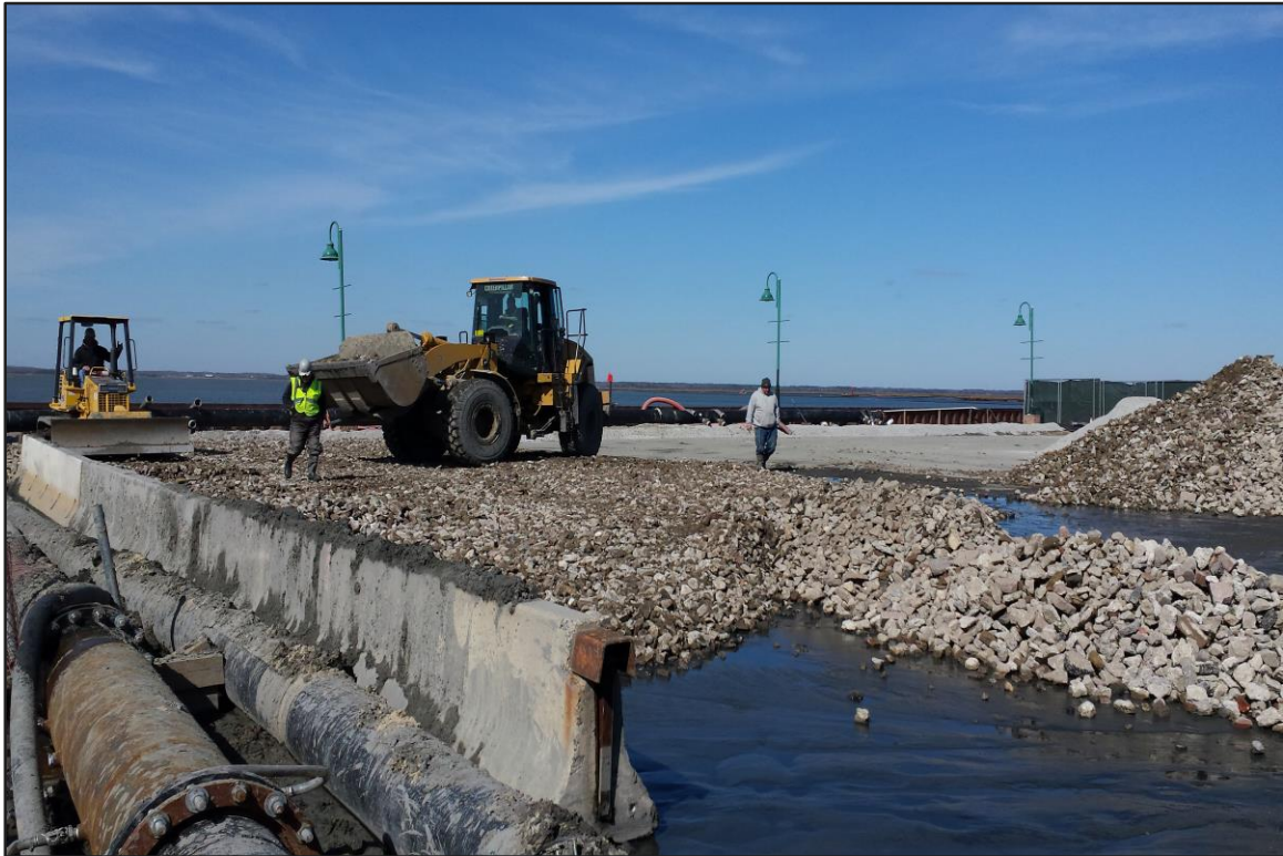
Photograph 13: De-watering Area – Pad preparation for geobags #5-9. (Looking northwest)
