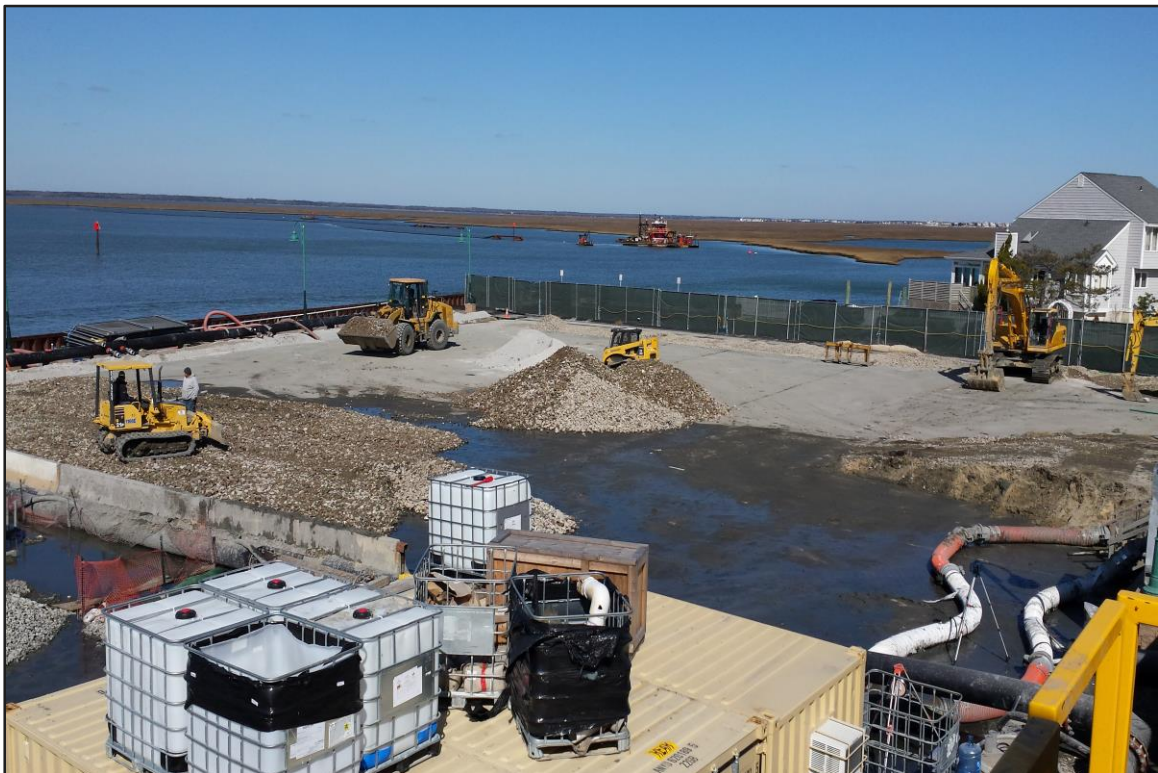
Photograph 8: De-watering Area – Pad preparation for geobags #6-9. (Looking northwest)
