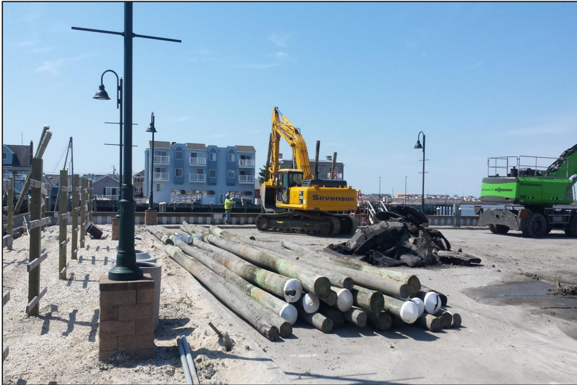
Photograph 7: De-Watering Area – Marina pile replacement in progress. (Looking south)
