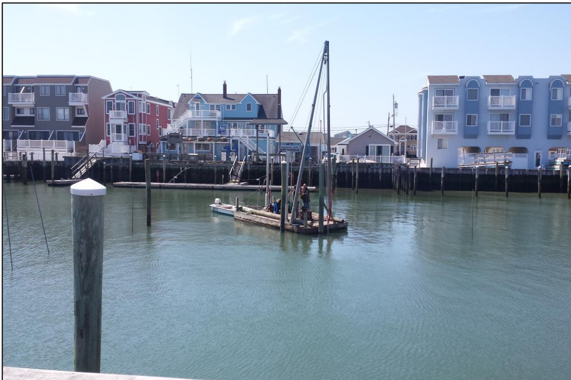
Photograph 8: North Basin – Marina pile replacement in progress. (Looking south)
