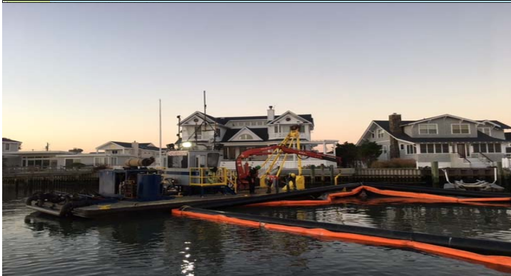
1 Tender boat assisting with curtain repair before dredging operations in Snug Harbor
