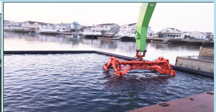
6 Clamshell Bucket going for dredge material inside of moon pool in Snug Harbor
