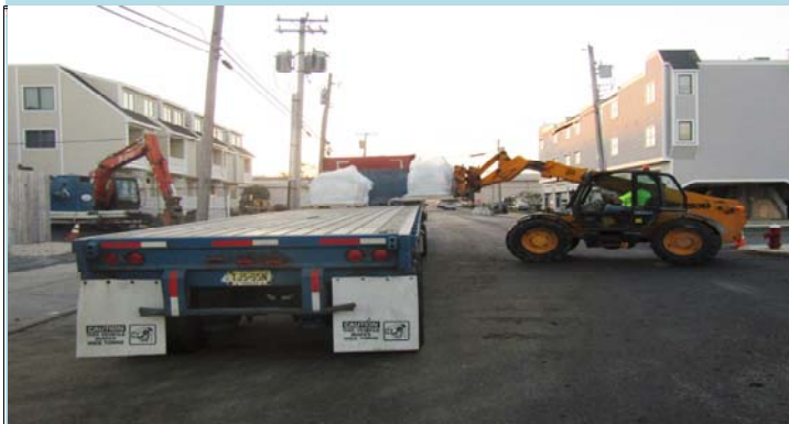
5 Unloading a truck of portland cement for blending operations
