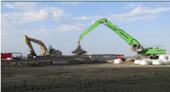
3 Blending dredge material with portland cement
