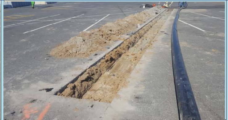
2 Completed excavation of drainage channel
