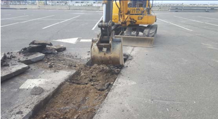
1 Excavating a drainage channel at the staging area
