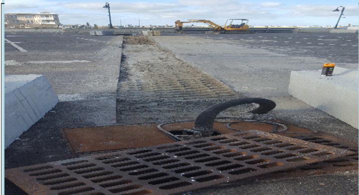
3 Backfilled channel and installed sump, channel prepped for paving
