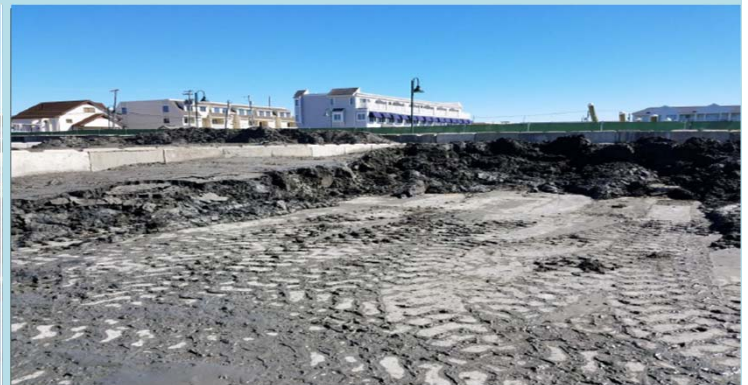
6 Stockpiling dredge material blended with Portland
