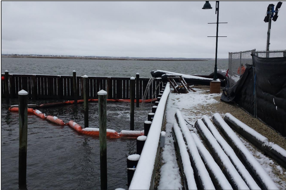
Photograph 9: North Basin/De-watering Area – Discharge pipes. (Looking west)
