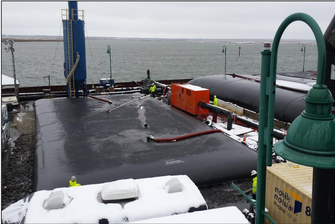
Photograph 5: De-watering Area – New geobag placed between #5 and #6. (Looking west)
