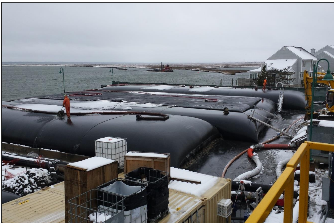
Photograph 6: De-watering Area – Geobags #6-#9 with an additional bag straddling #7-#8. (Looking north)
