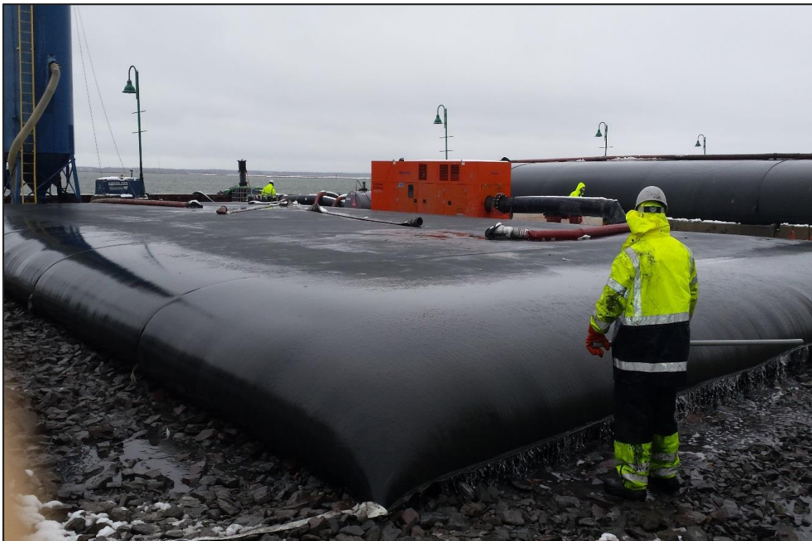
Photograph 8: De-watering Area - New geobag placed between #5 and #6. (Looking west)
