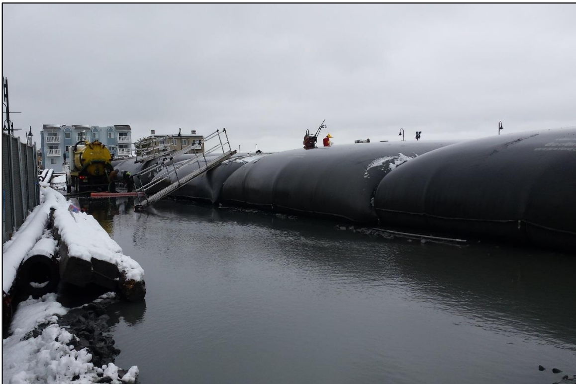
Photograph 10: De-watering Area – Geobags #1-#5. (Looking south)
