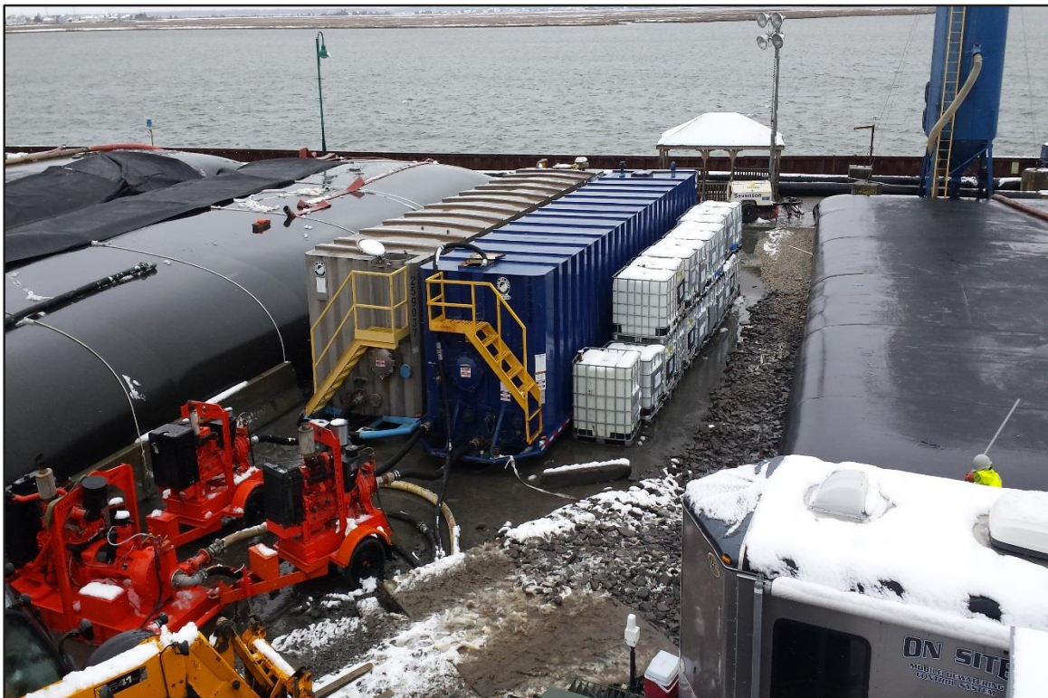
Photograph 4: De-watering Area – Pumping equipment in operation. (Looking west)
