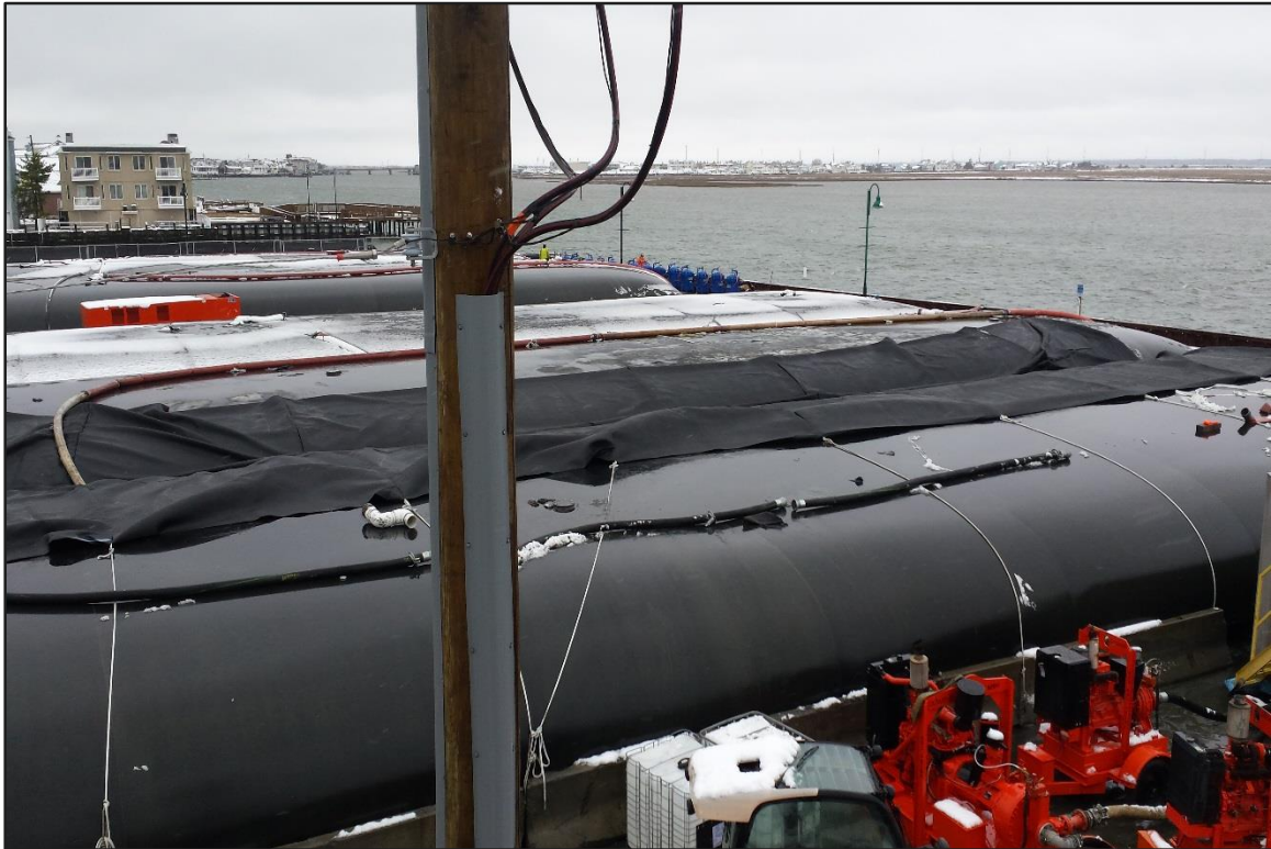
Photograph 3: De-watering Area – Geobags #1-#5 with an additional bag straddling #4-#5. (Looking south)
