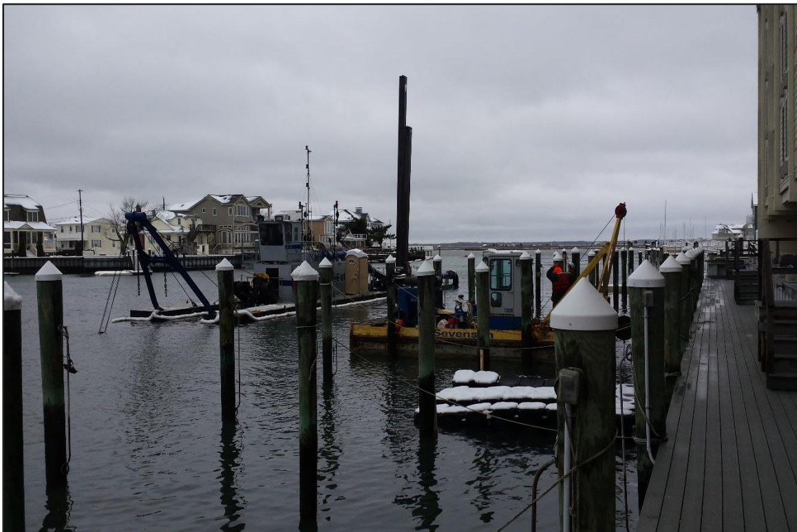
Photograph 12: Shelter Haven – Hydraulic dredge and support boat. (Looking west)
