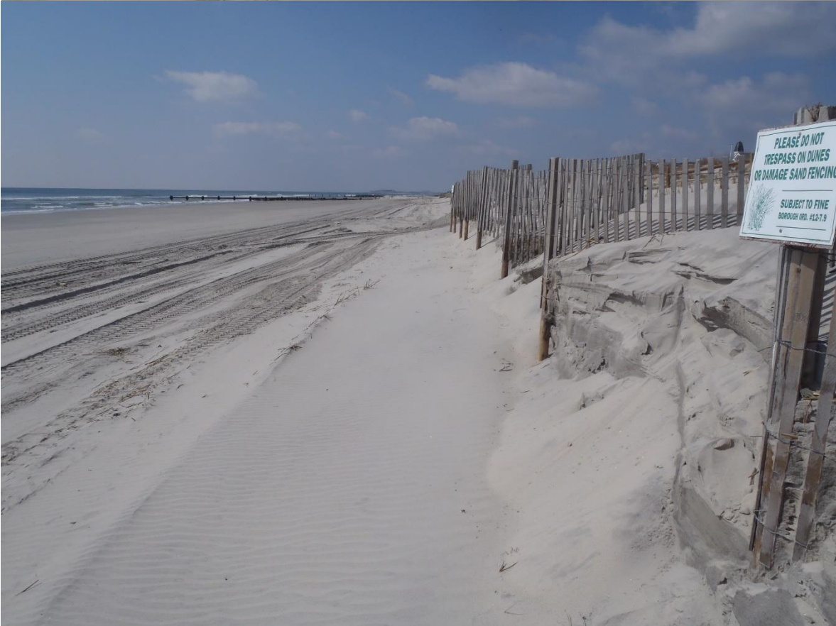
Photoplates 5a & b – The photo taken April 10, 2018 is in sharp contrast with those four sites to the north. Here the dune toe was eroded to the fence installation compromising some fence sections. The beach is very flat and much narrower than in June or October 2017.
