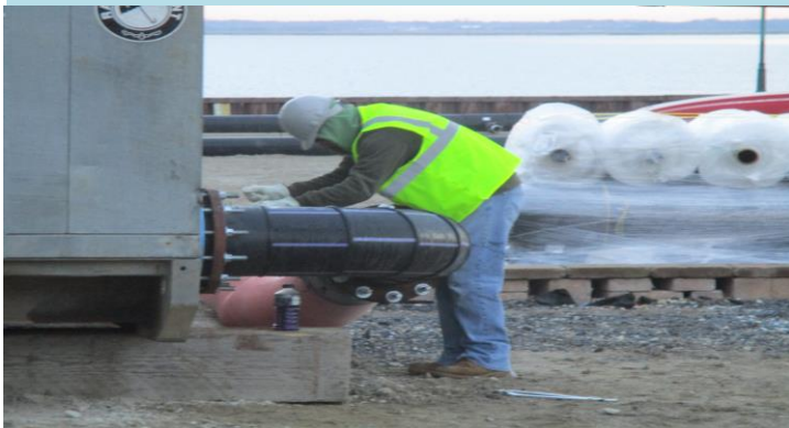
3 Tightening flange on the discharge side of Rain for Rent pump.
