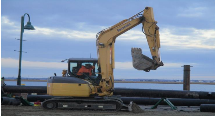
1 Grading the process pad.
