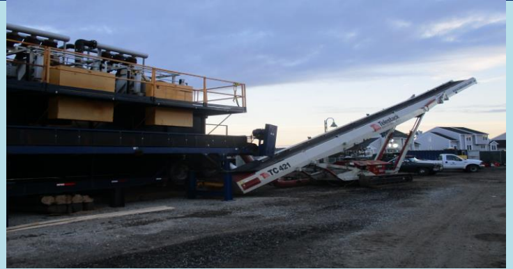
2 Placed the stacking conveyor into position.
