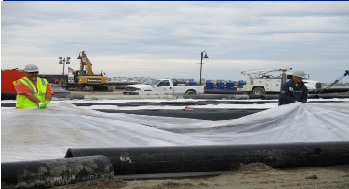
1 Pulling poly on the south process pad.
