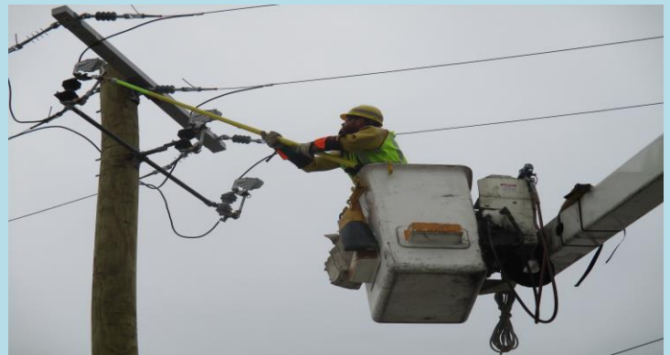
4 Atlantic City Electric activating power.
