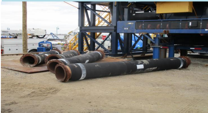
5 Dredge hose delivered to site.
