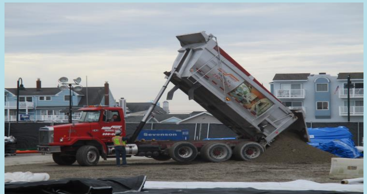
6 Action Supply delivering dense grade aggregate to the site.
