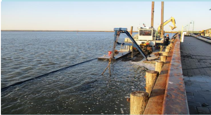
3 Shark dredge positioned against the bulkhead.
