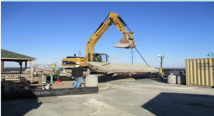
5 Transporting crane mats.
