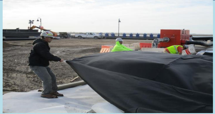
2 Continuing to deploy Geotubes in the south process area.
