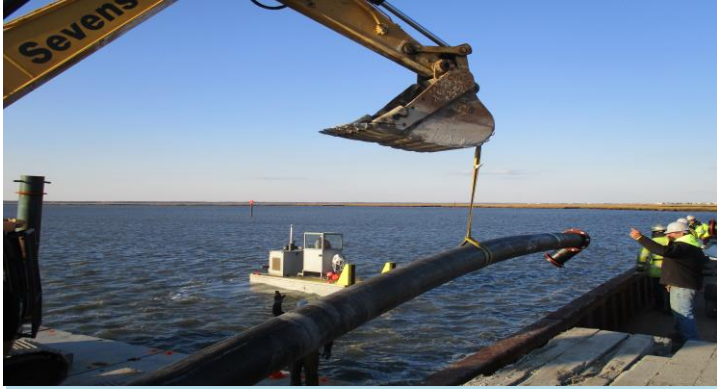
1 Placing HDPE with the excavator positioned on the barge.
