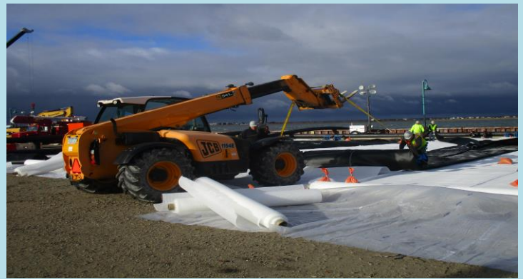
4 Continuing to roll out geotubes with forklifts.
