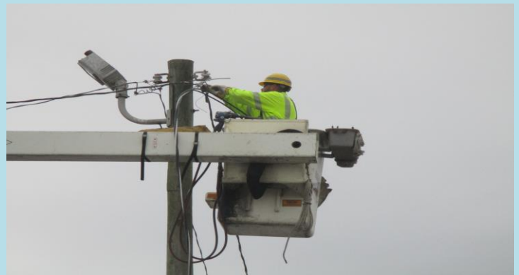
6 Atlantic City Electric installing the electrical drop to the office trailers (11/12/15)
