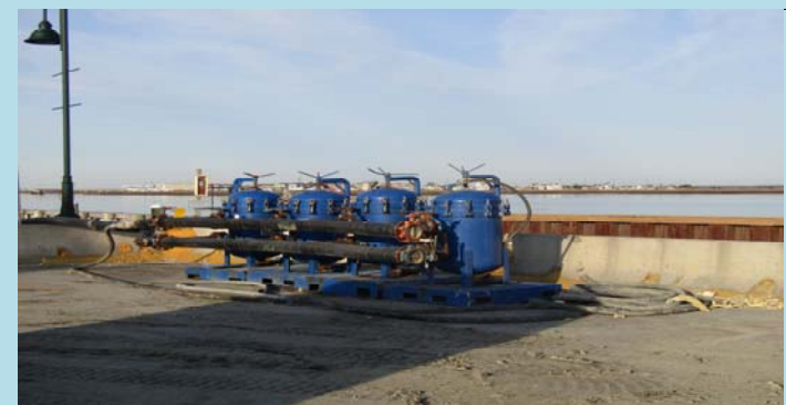
6 Breaking down the water treatment system
