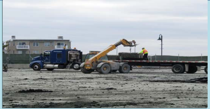
2 Loading a truck with bin blocks
