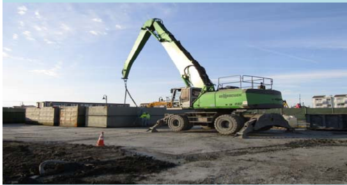
3 Sennebogen picking scows out of the water for demob
