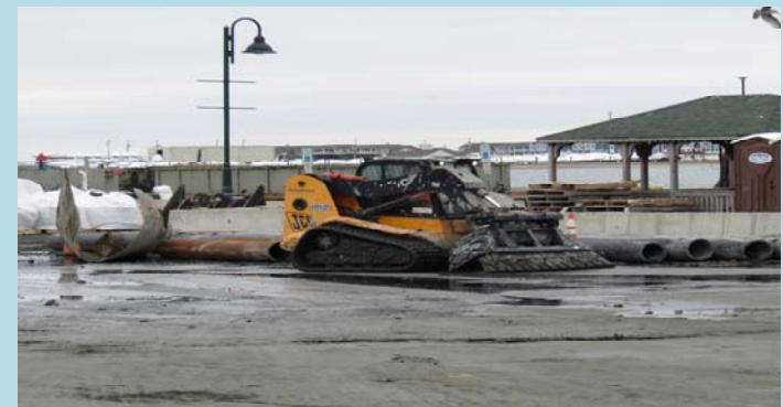
4 Cleaning the North pad with a JCB skid steer
