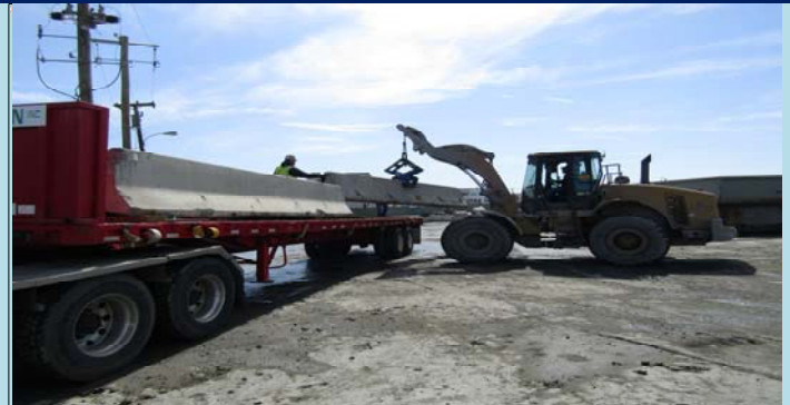
2 Loading a truck with Jersey Barriers
