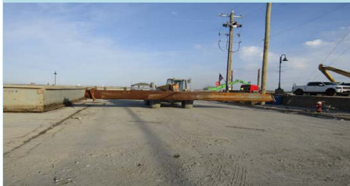
3 30' spuds taken off the PC-400 barge for demob
