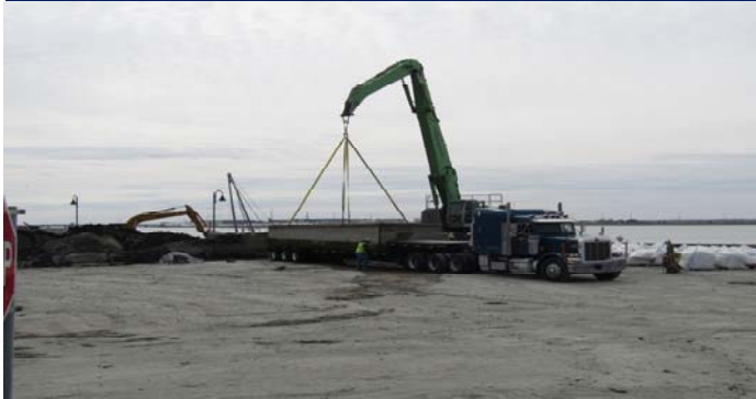
1 Loading a truck with a 40' float to be taken off site
