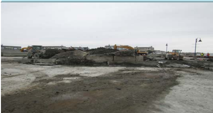
5 Breaking down the mixing cells on the South pad
