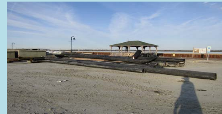
6 HDPE pipe ready to be taken off site
