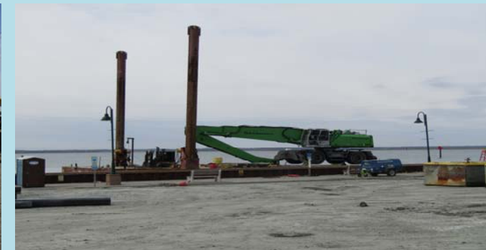
4 Sennebogen barge ready to be taken to Northstar Marine for Demob
