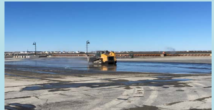
4 JCB skid steer cleaning the North pad
