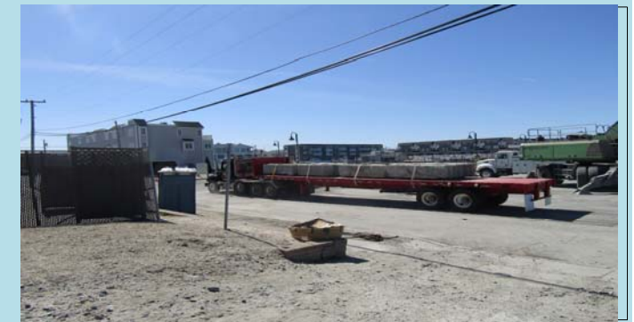
6 Load of bin blocks being taken off site
