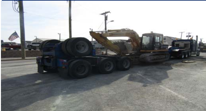
1 Loading a Cat 312 excavator for demob
