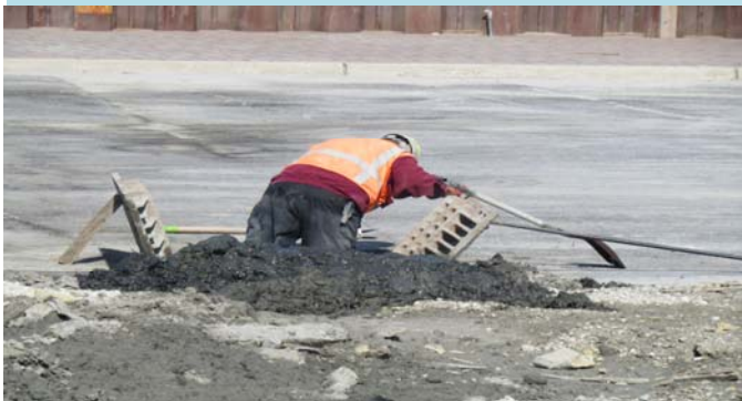
3 Repairing sump on the South pad
