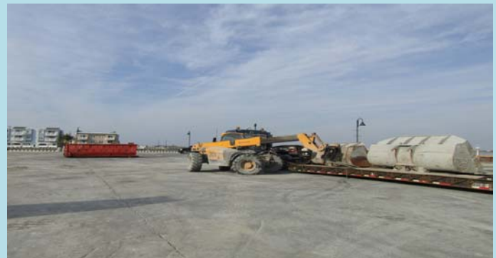
4 JCB loading two buckets on a truck
