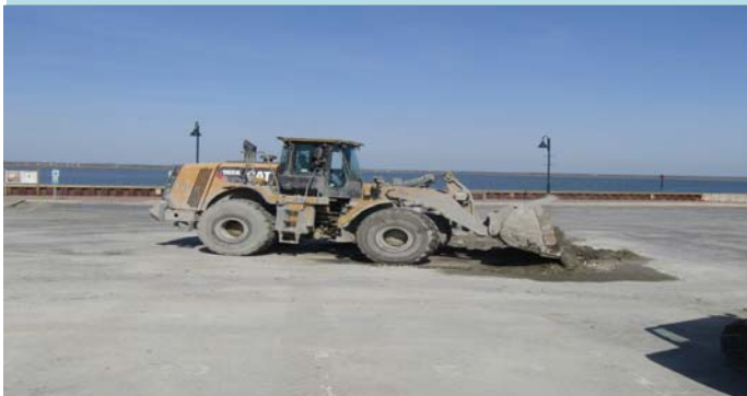
5 Loader finishing sump repairs
