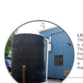
**LOCATION:** Clark, NJ This cistern was installed at a public works department. The rainwater is harvested from the rooftop of the building and used as part of a "green car wash" system that uses rainwater.
