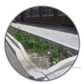
**LOCATION:** Camden, NJ This stormwater planter was designed to capture stormwater runoff from the street in front of the Brimm School in Camden, New Jersey. **CURB CUT** This curb cut and concrete flow pad are
