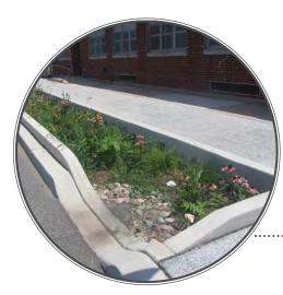
**LOCATION:** Camden, NJ This stormwater planter was designed to capture stormwater runoff from the street in front of the Brimm School in Camden, New Jersey. **CURB CUT** This curb cut and concrete flow pad are designed to help redirect stormwater runoff to the rain garden system and
