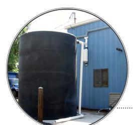
**LOCATION:** Clark, NJ This cistern was installed at a public works department. The rainwater is harvested from the rooftop of the building and used as part of a "green car wash" system that uses rainwater.
