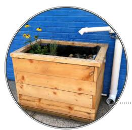
LOCATION: Camden, NJ Downspout planters are installed at the end of a downspout to capture, store, and slowly discharge stormwater back to the nearest storm sewer system.
